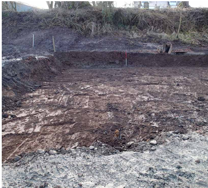
Fig. 4 - Development area with steep slope below burial ground in background
