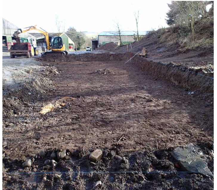
Fig. 3 - Development area from NW following groundworks
