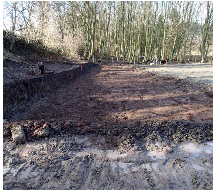
Fig. 5 - Development area from SE following groundworks
