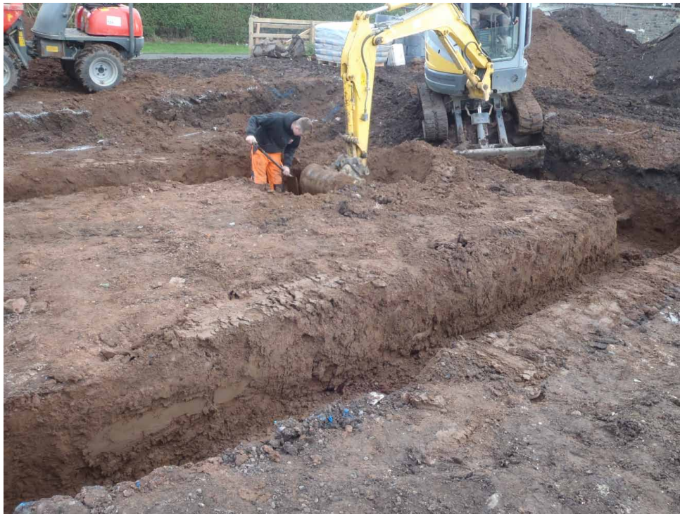
Fig. 2 - Working shot and general view of site
