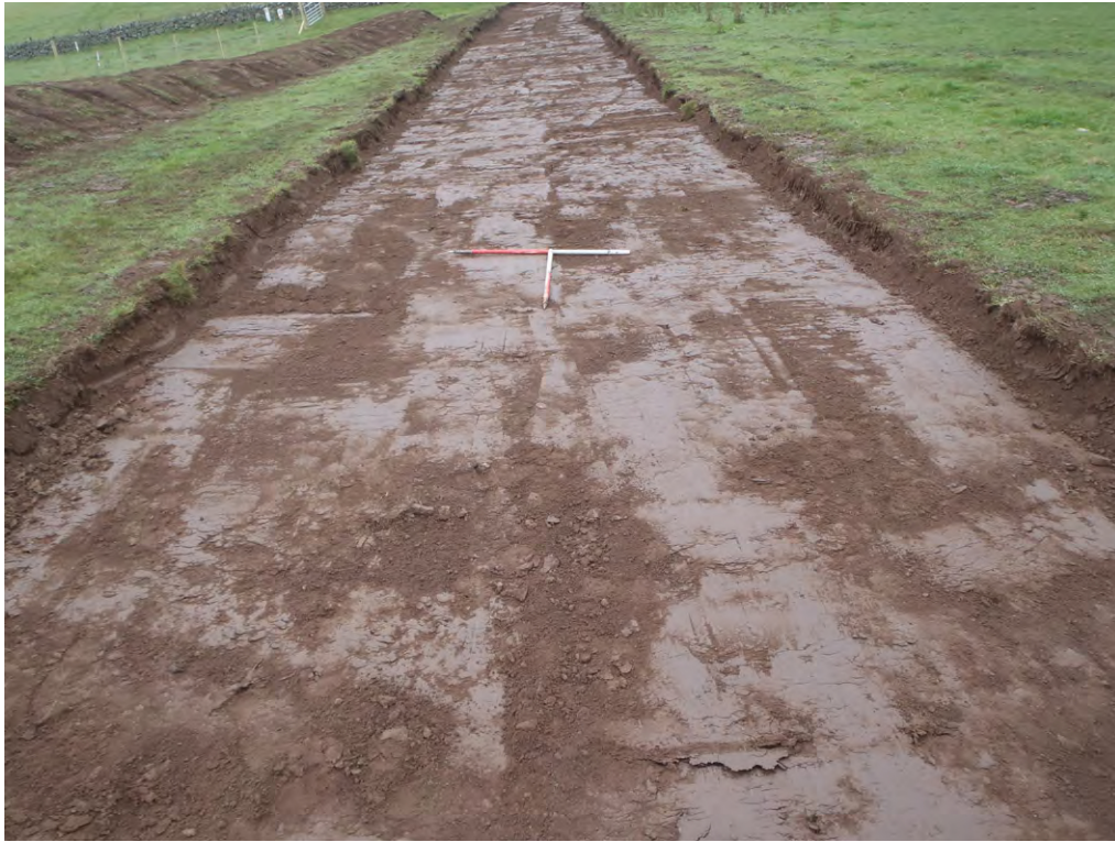
Fig. 6 Initial topsoil strip exposed to subsoil depth
