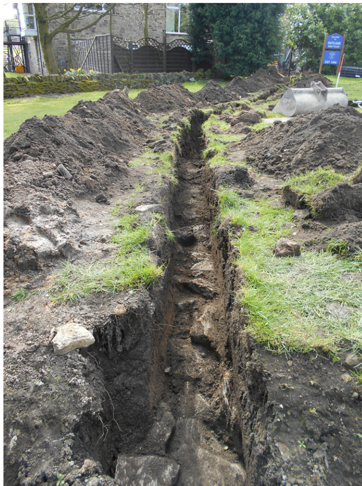
Fig. 17 - Shot of service trench after topsoil removal with possible rampart footing 039
