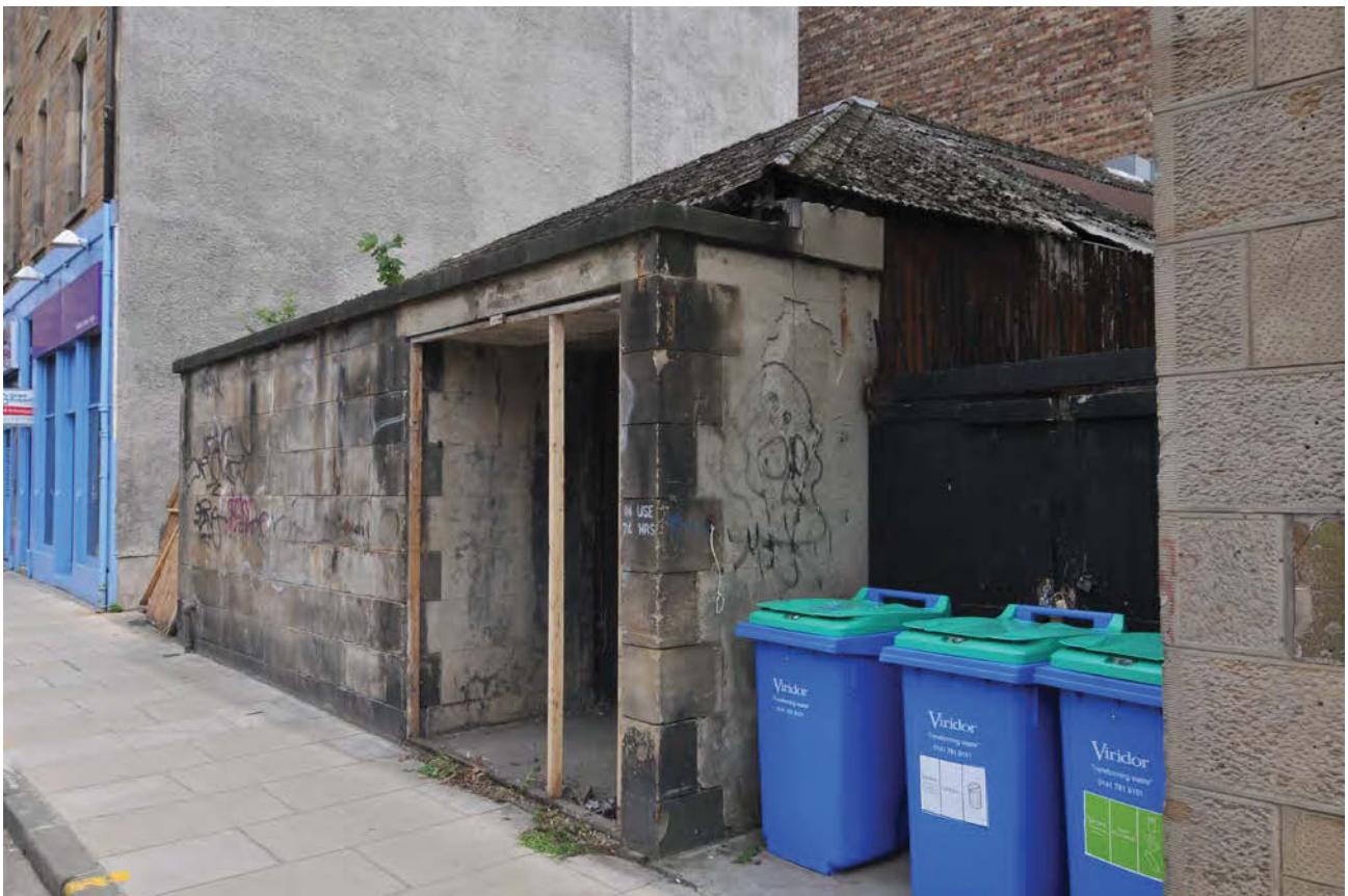
Plate 22. Oblique view of queue shelter
