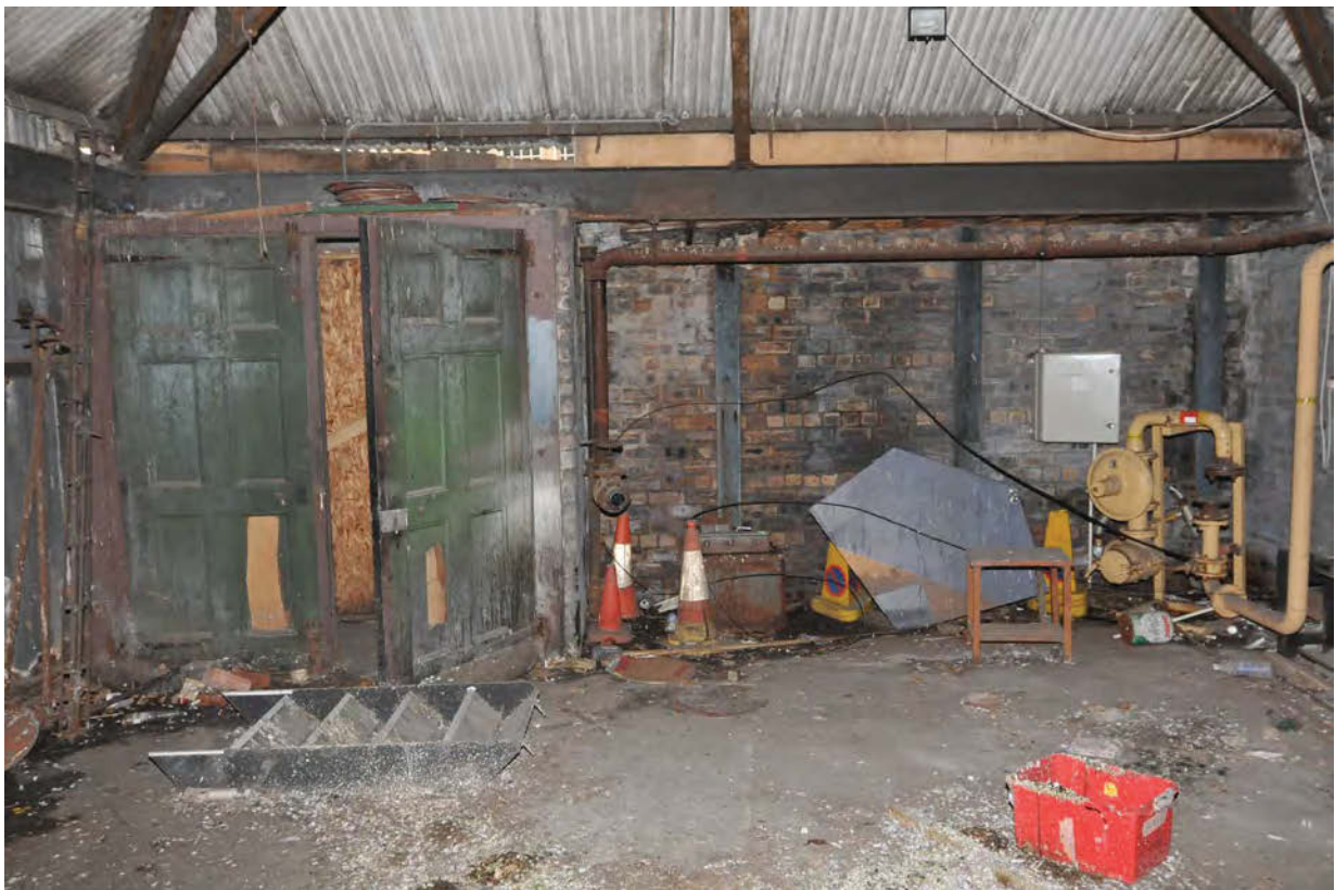
Plate 4. Internal east-facing elevation of the queue shelter
