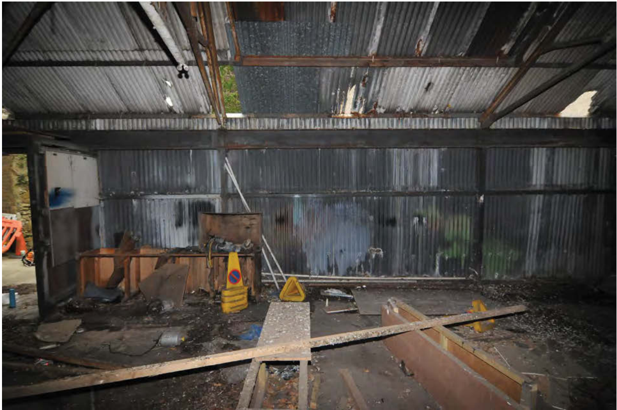
Plate 6. Interior north-facing elevation of the queue shelter showing its steel frame
