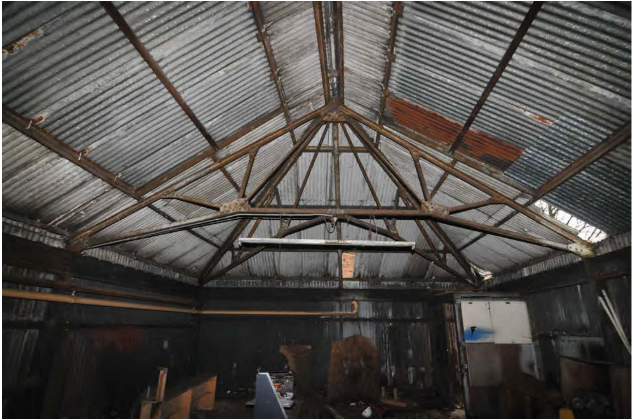
Plate 7. Composite angle-iron truss detail
