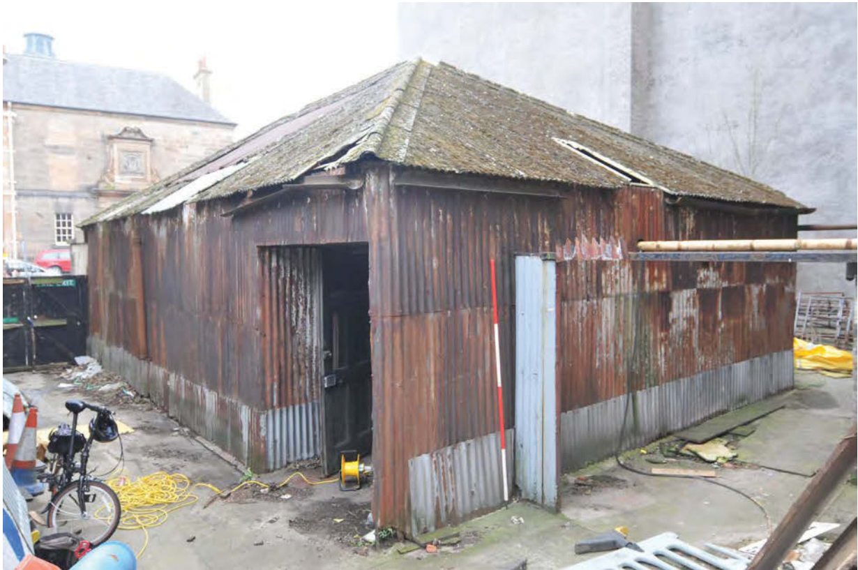
Plate 2. Rear and south-facing elevation of the queue shelter
