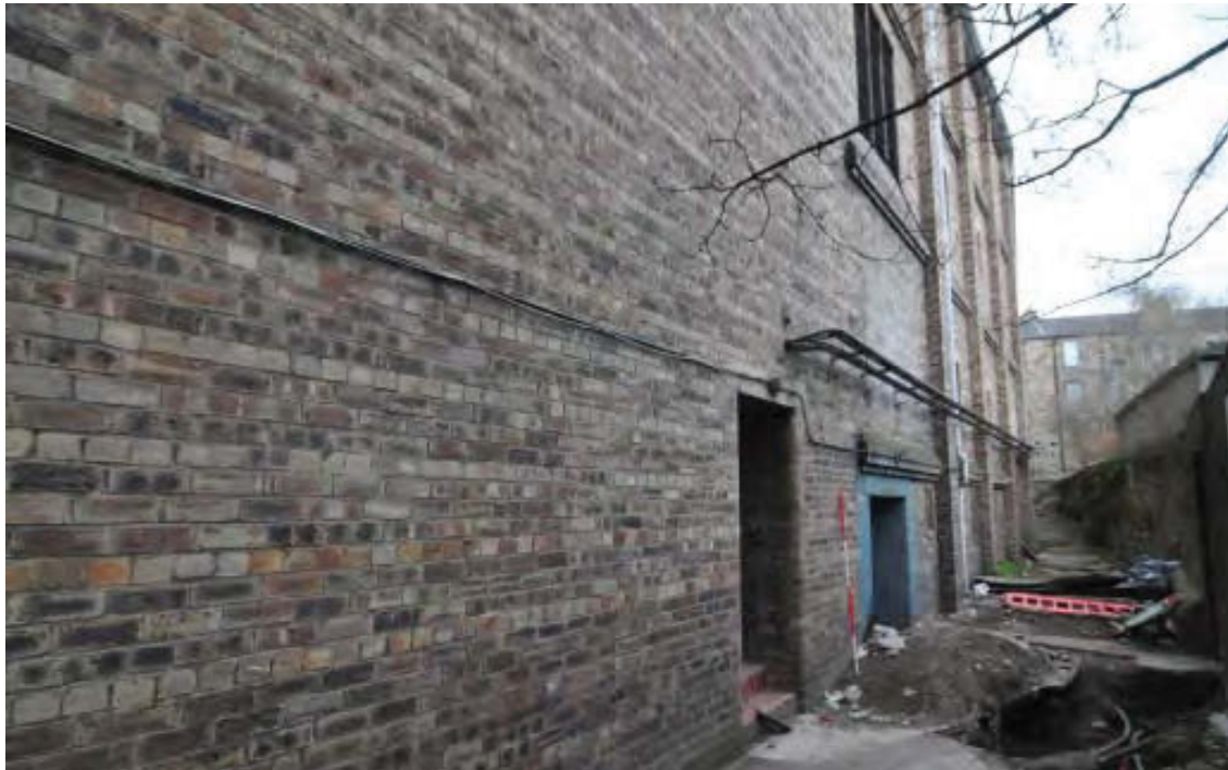
Plate 13. Oblique view of south-facing elevation of Fly Tower
