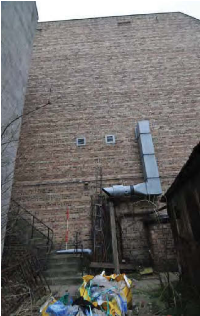
Plate 9. Central part of west-facing elevation of Fly Tower
