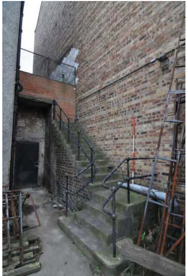
Plate 10. Detail of stairs, west-facing elevation of Fly Tower
