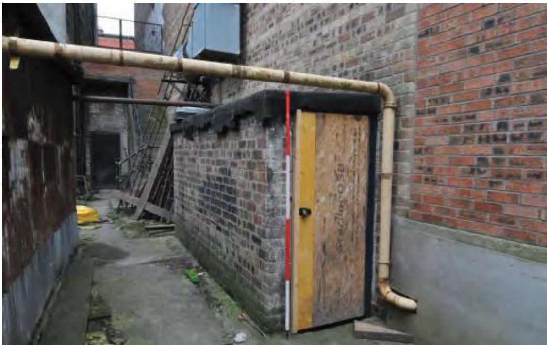
Plate 11. Detail of shed, west-facing elevation of Fly Tower
