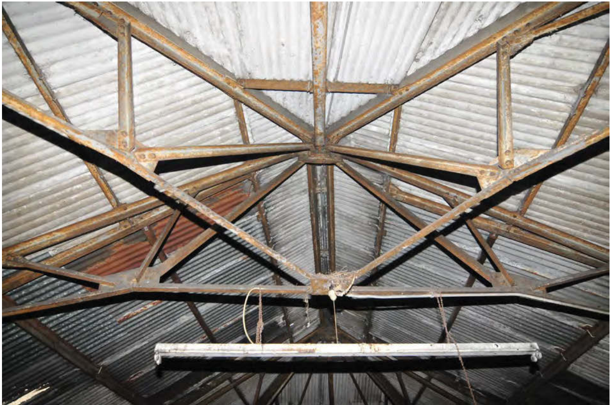
Plate 8. Hip truss projecting of the main pitched truss
