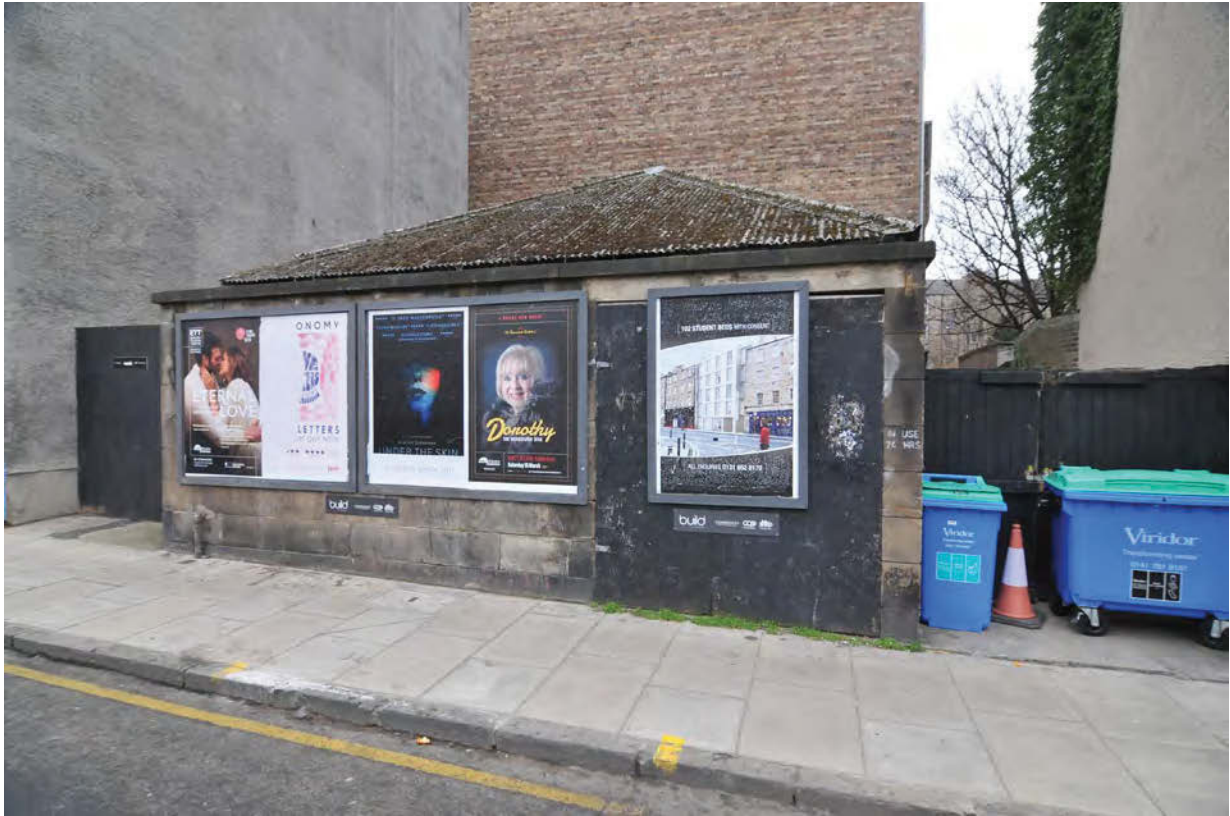
Plate 1. Street-front west-facing elevation of the queue shelter
