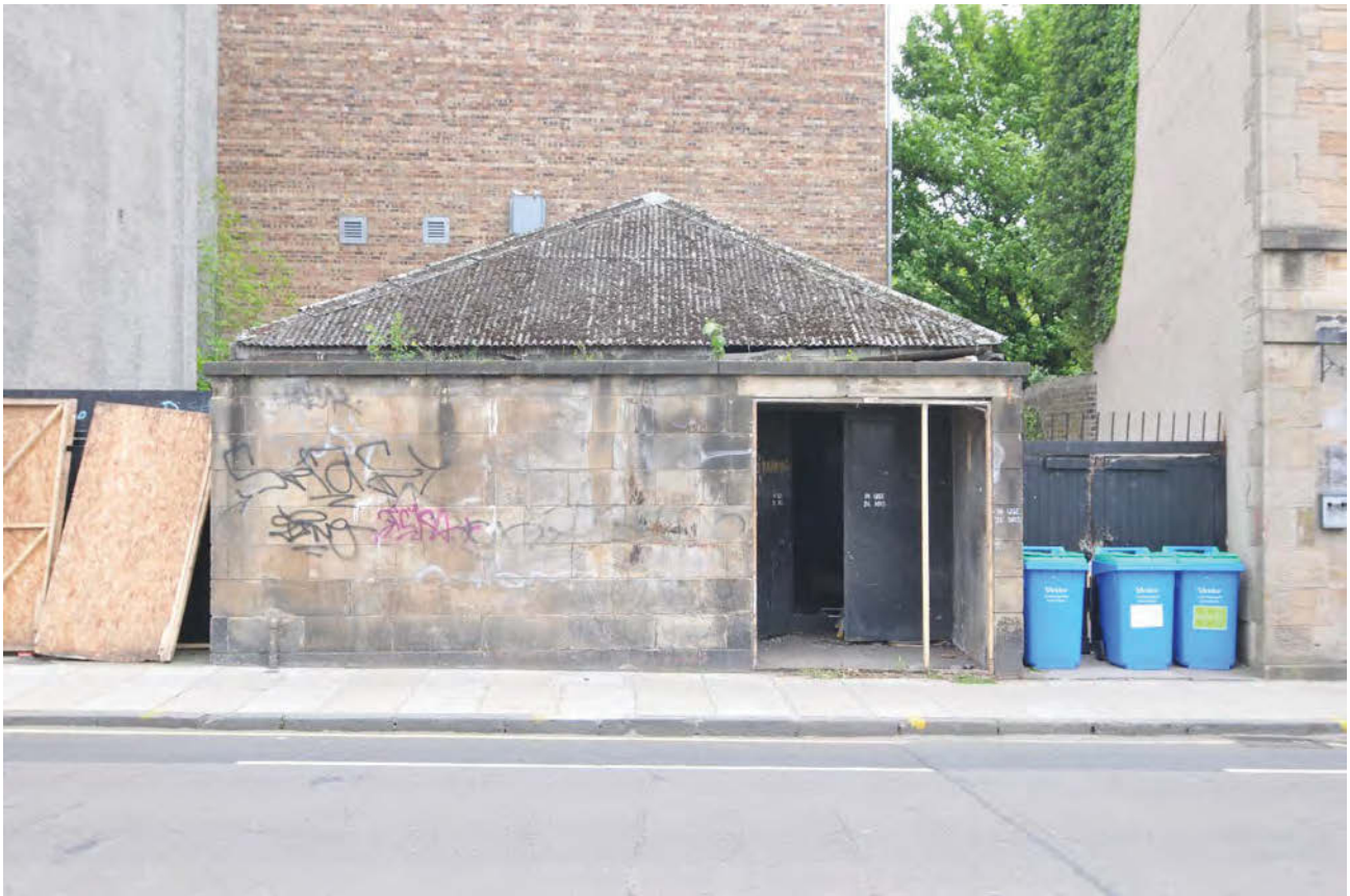
Plate 21. West-facing elevation of Queue Shelter
