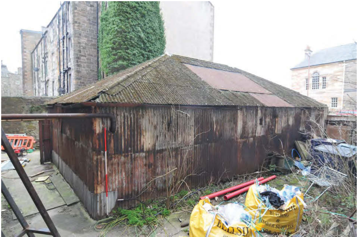
Plate 3. Rear and north-facing elevation of the queue shelter
