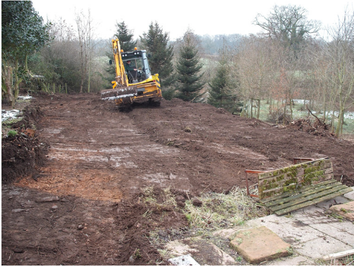
Fig. 2 - General shot of Phase 1 Watching Brief after topsoil stripping
