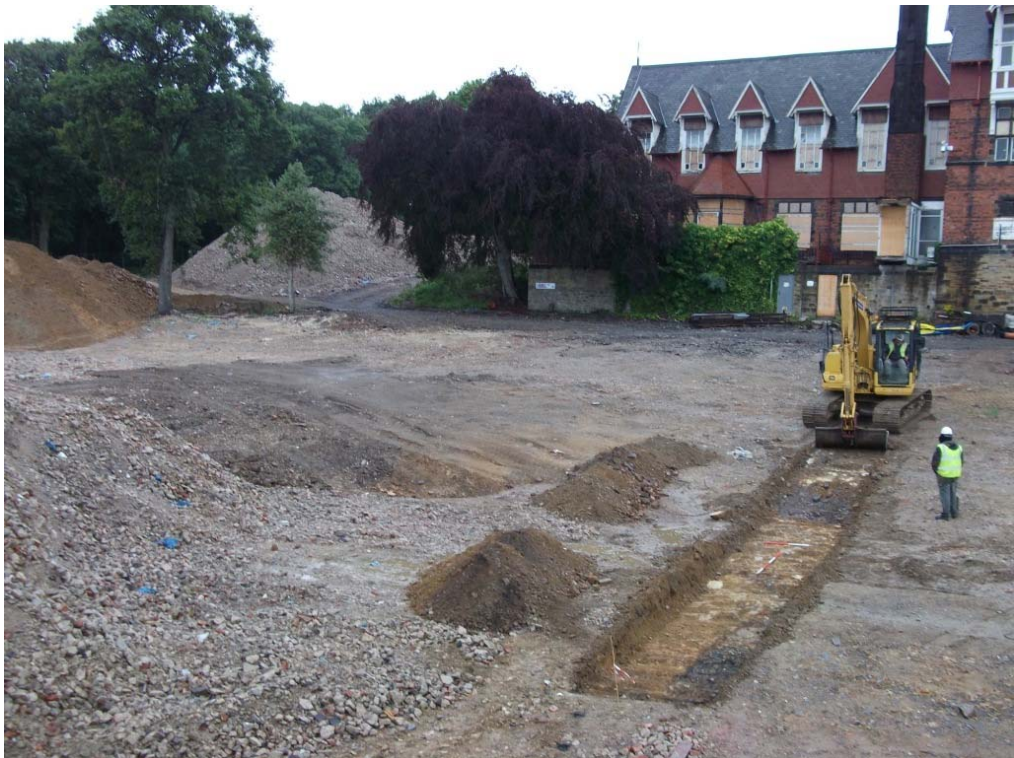
Plate 15: Working Shot, Excavation of Trench 4 Looking North
