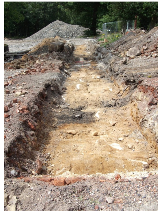
Plate 8: Trench 8 Looking Northwest
