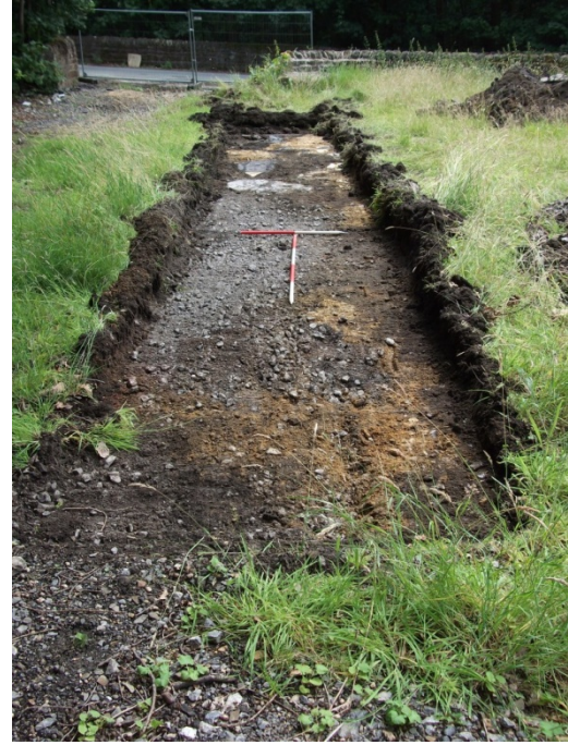
Plate 12: Trench 12 Looking Southeast
