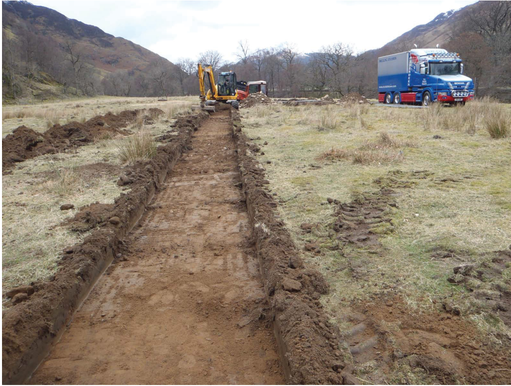
Fig. 2 - Cable trench from SE
