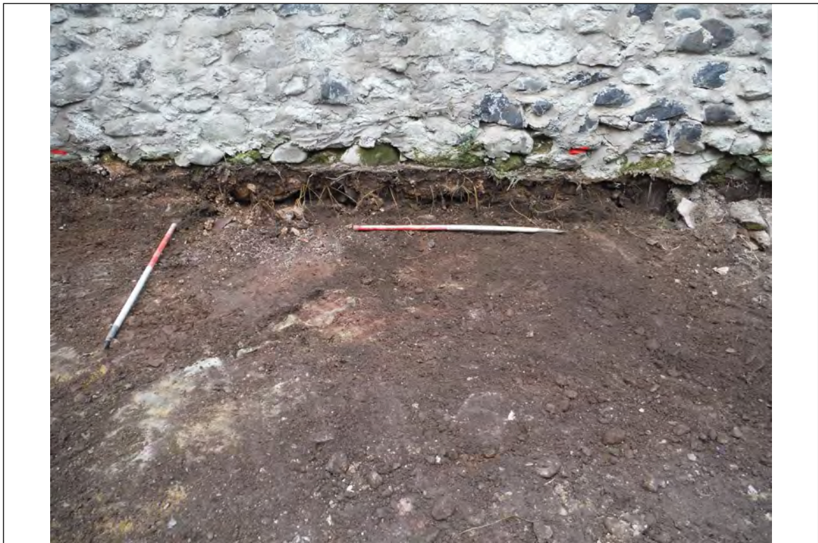
Plate 18 – Wall founded on natural river gravels (007)
