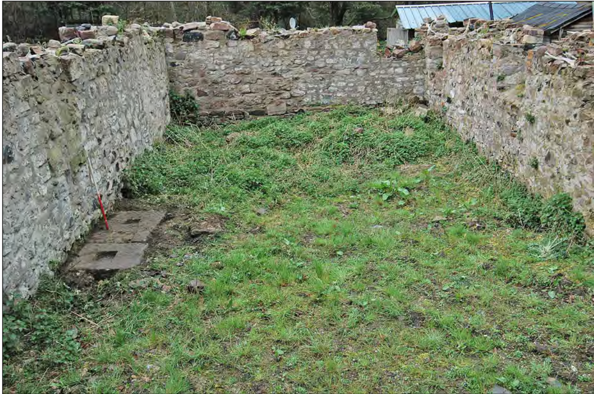
Plate 13 – Hurst plinths in relation to the building layout, looking north
