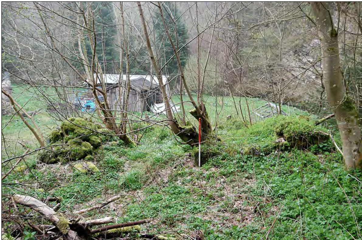
Plate 16 – Ruined building remains on the east side of the mill looking south
