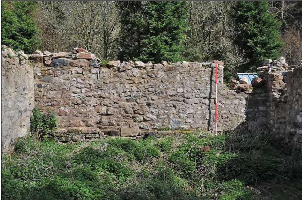
Plate 11 – Internal south-facing elevation
