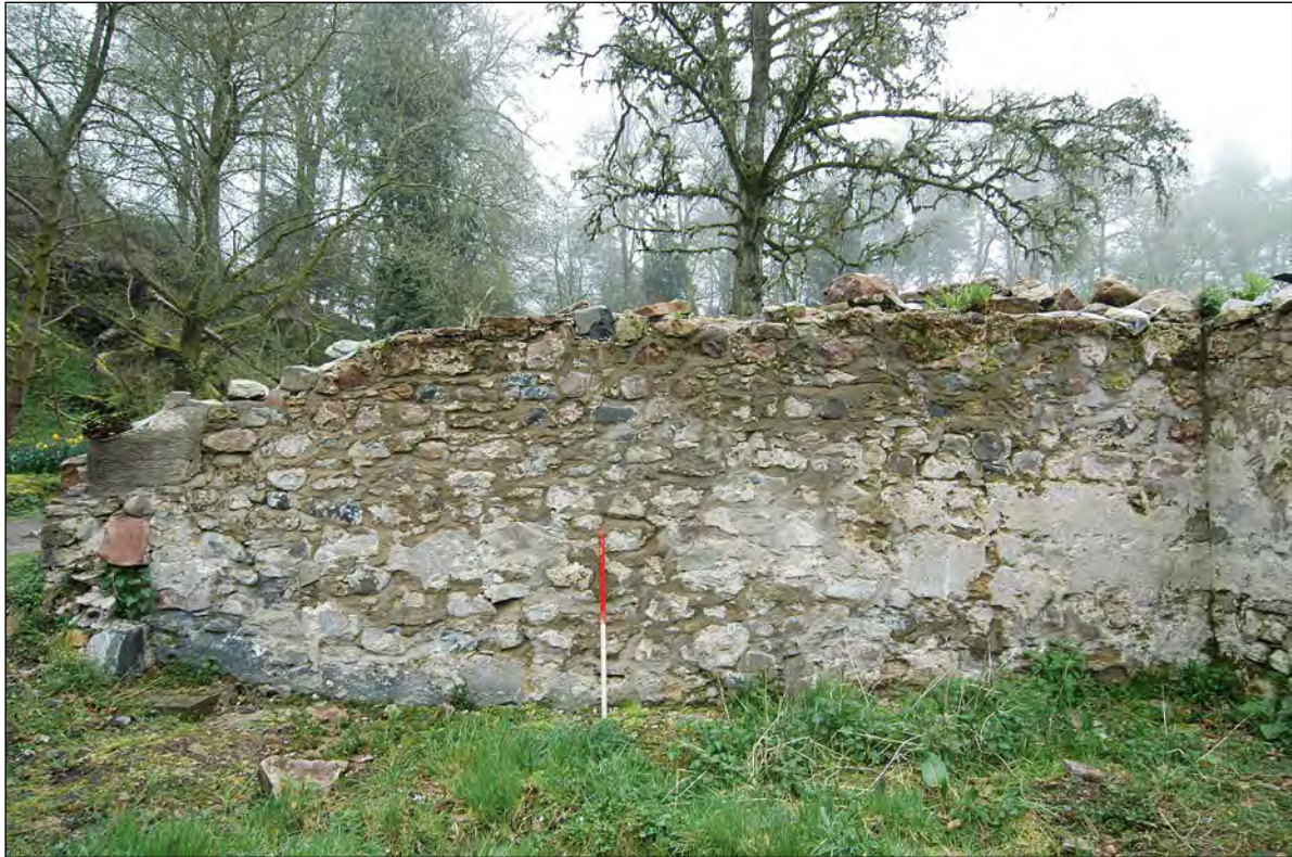
Plate 7 – Internal north-facing elevation
