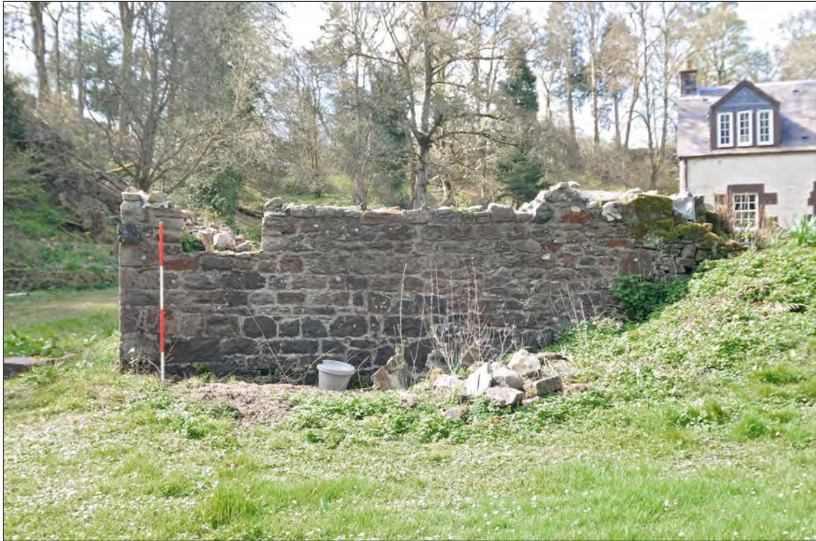
Plate 3 – External north-facing elevation
