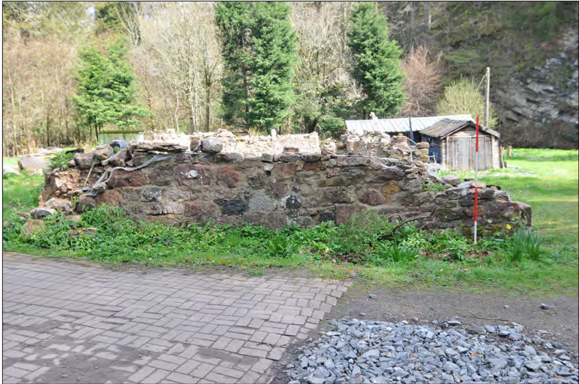
Plate 5 – External south-facing elevation
