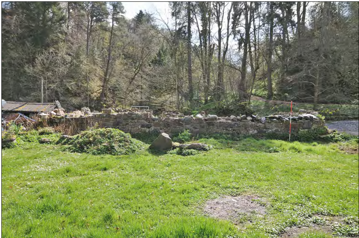
Plate 6 – External west-facing elevation
