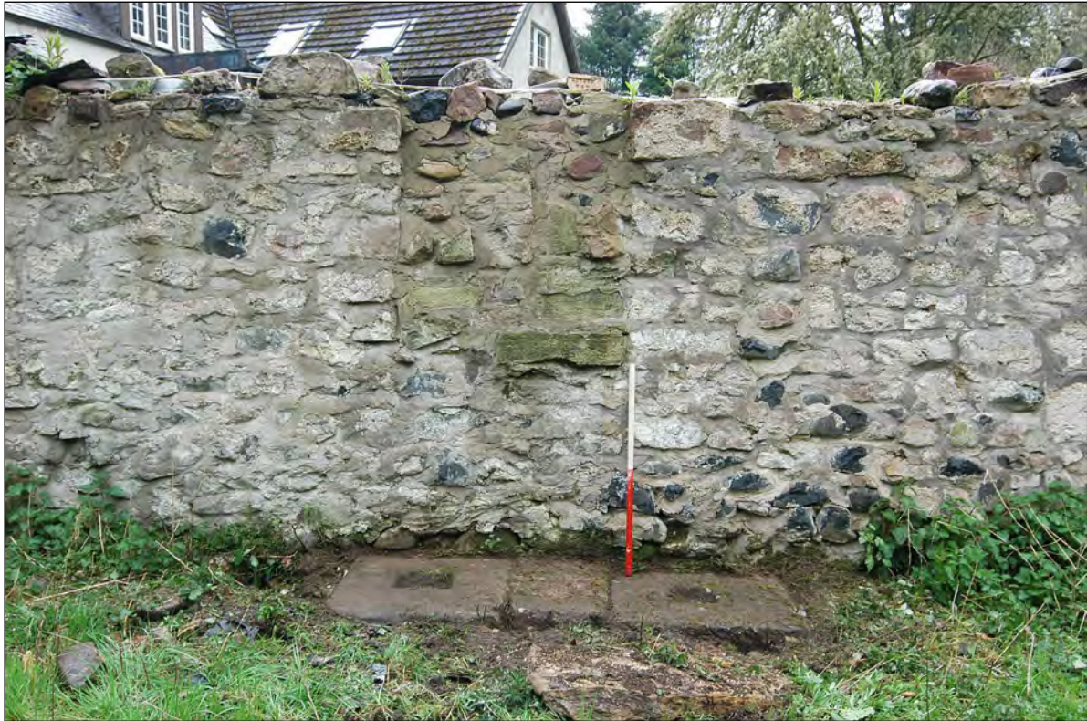
Plate 9 – Internal east-facing elevation (mid-section)
