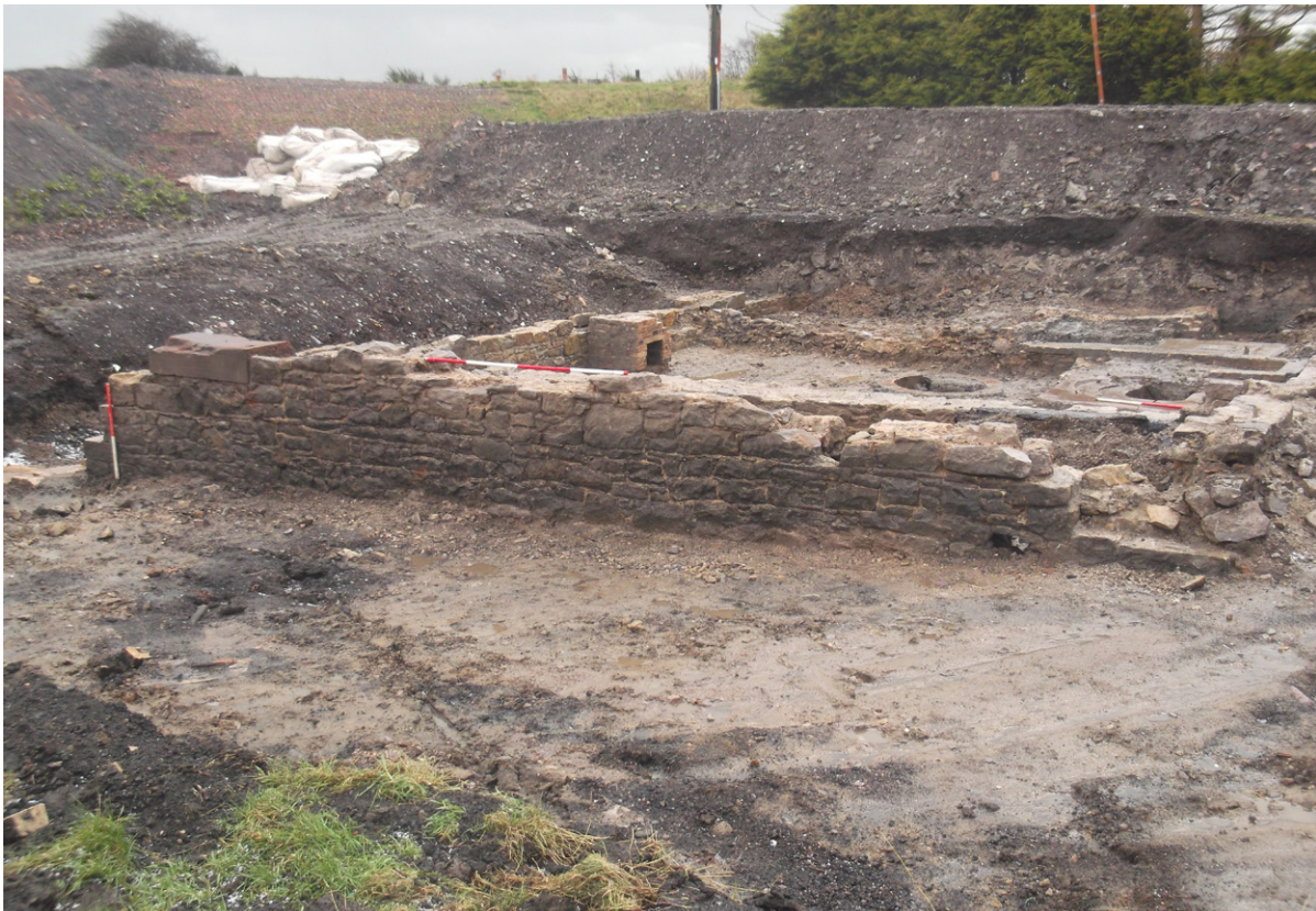
Plate 2: North-west facing elevation of Wall 124, Structure 1
