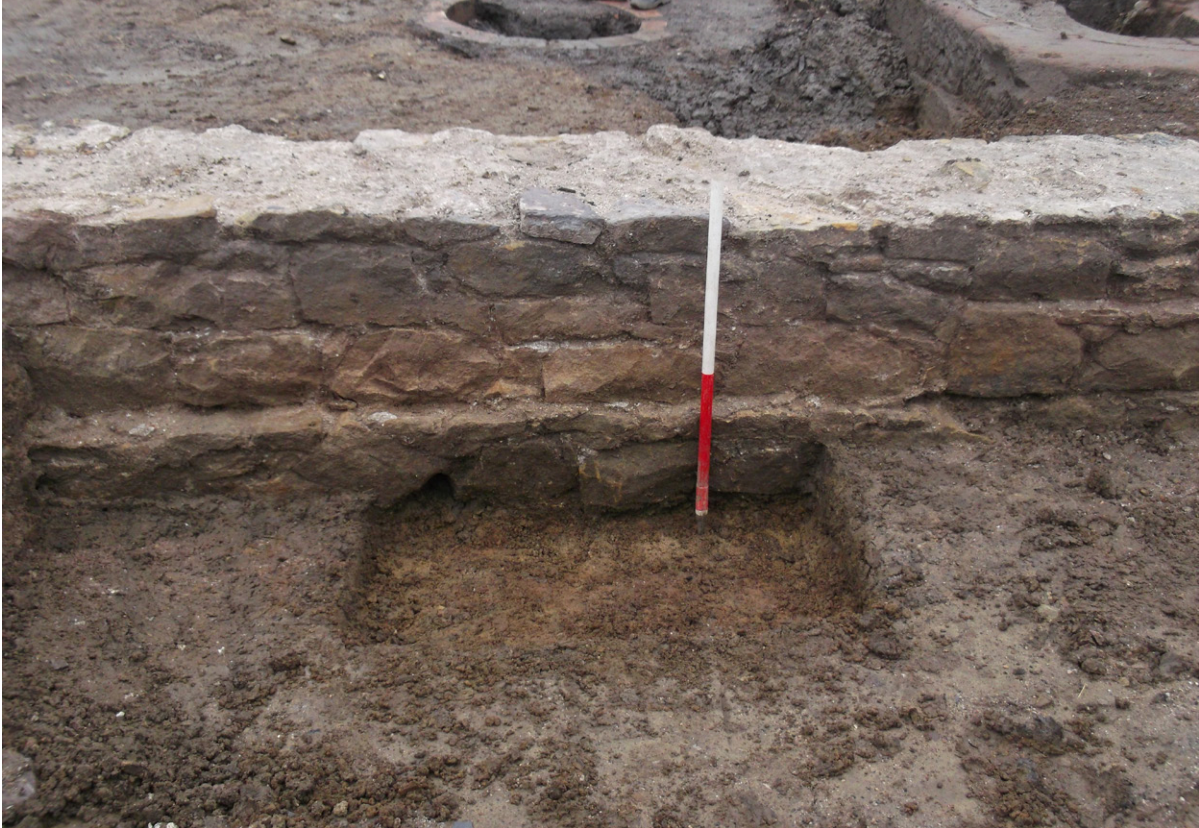
Plate 3: Foundations of north-west facing elevation of Wall 127, Structure 1
