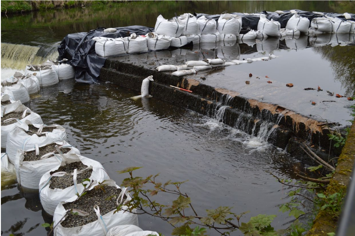
Plate. 5 - North-west-facing shot of Burley Mill Weir following damming of the river
