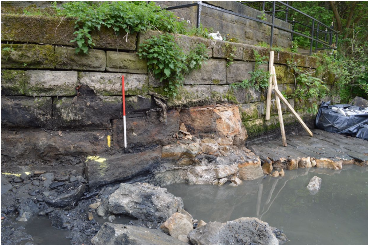
Plate. 7 - West-facing profile of Weir Head 103 following excavation
