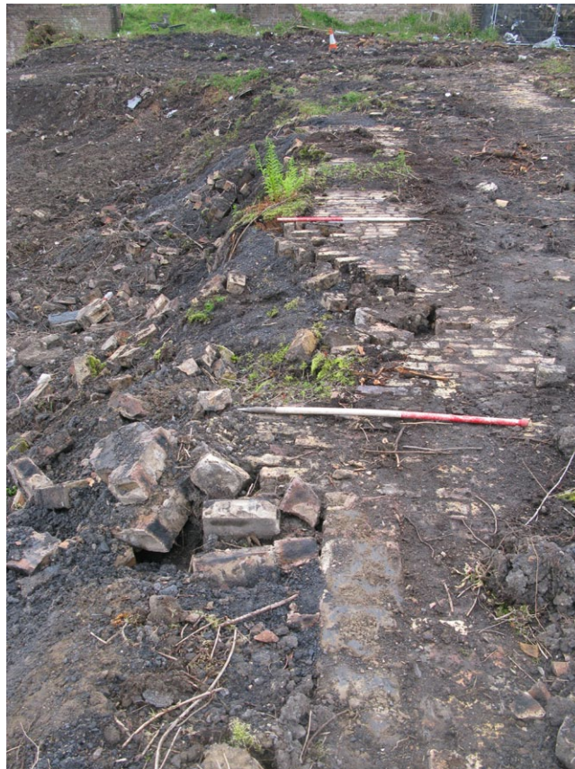
Fig. 15 - Shot showing where brick surface of platform extends out past the NE wall - possible 1st floor entrance to the factory, from the W
