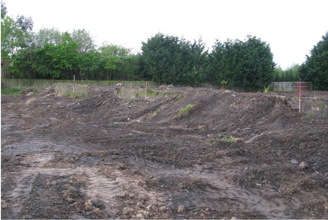
Fig. 12 - General shot of the platform, from the E
