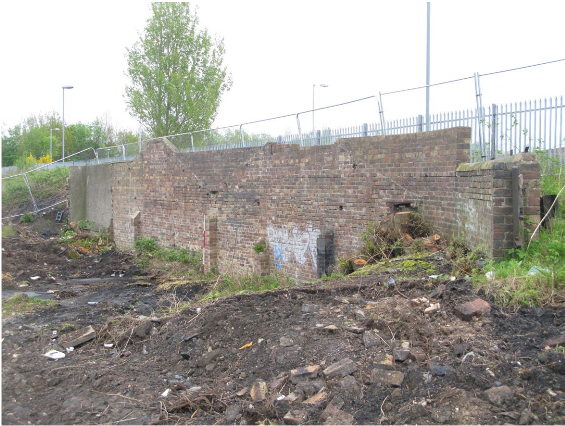
Fig. 14 - Shot of gable wall of double-roofed warehouse, from the SW
