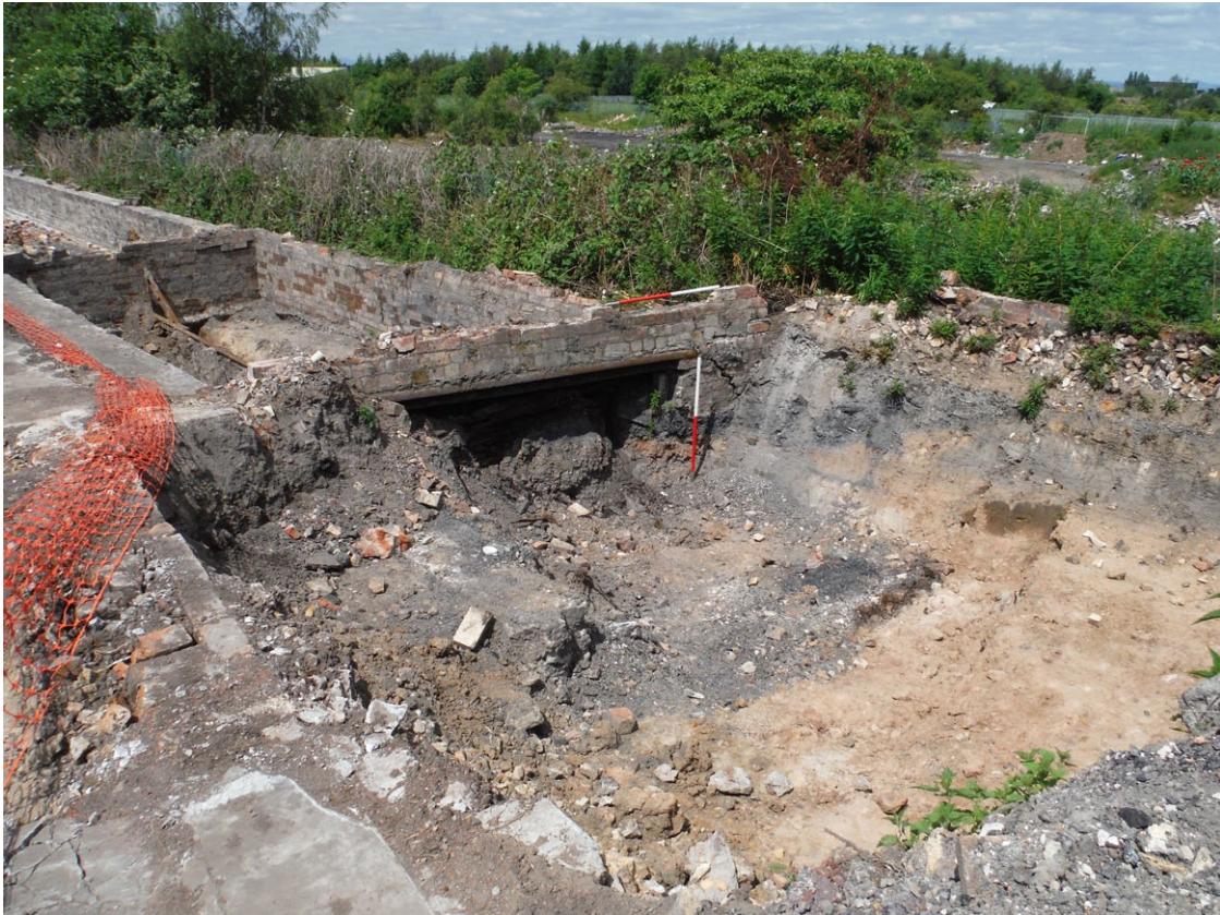
Fig. 22 - Building 4 from south-east
