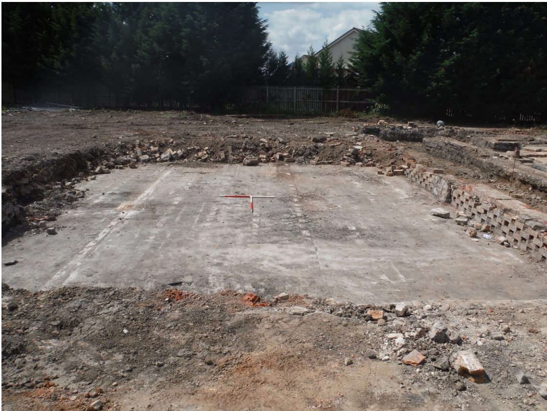
Fig. 12 - Building 1 from the east
