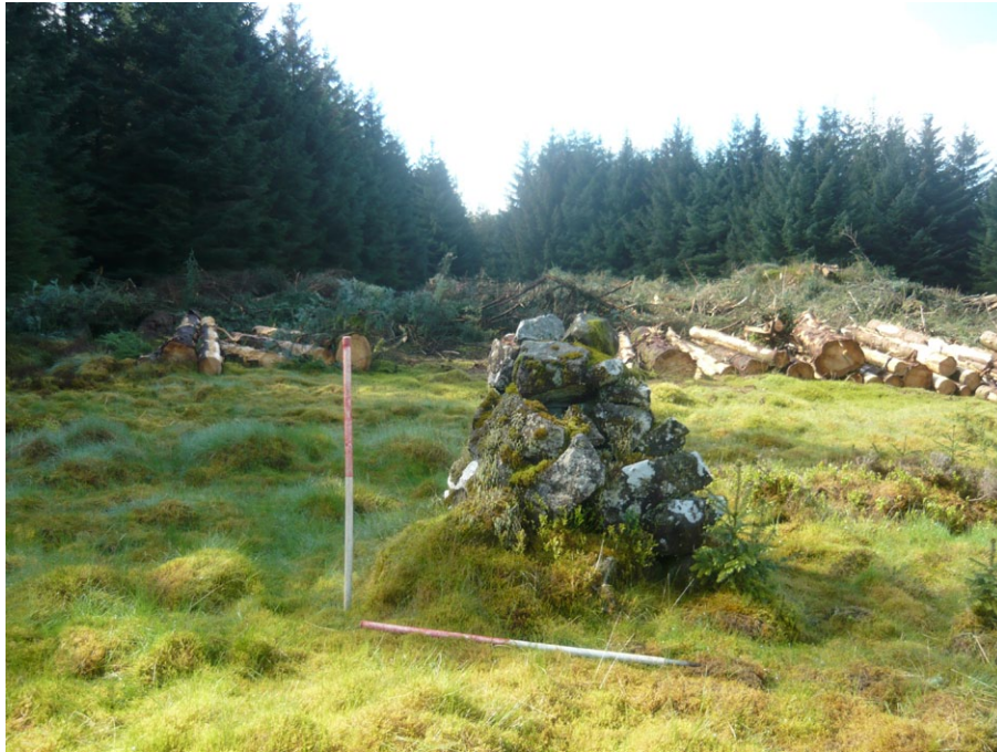
Fig. 2 - General shot of Shepherds Cairn (Site 13) prior to its deconstruction
