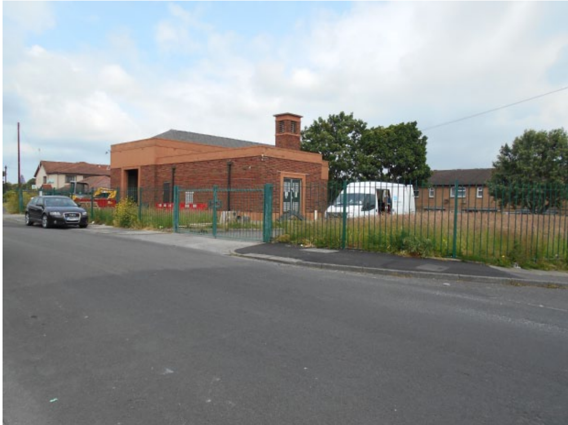
Plate. 1 - Pumping Station at Lennox Gate
