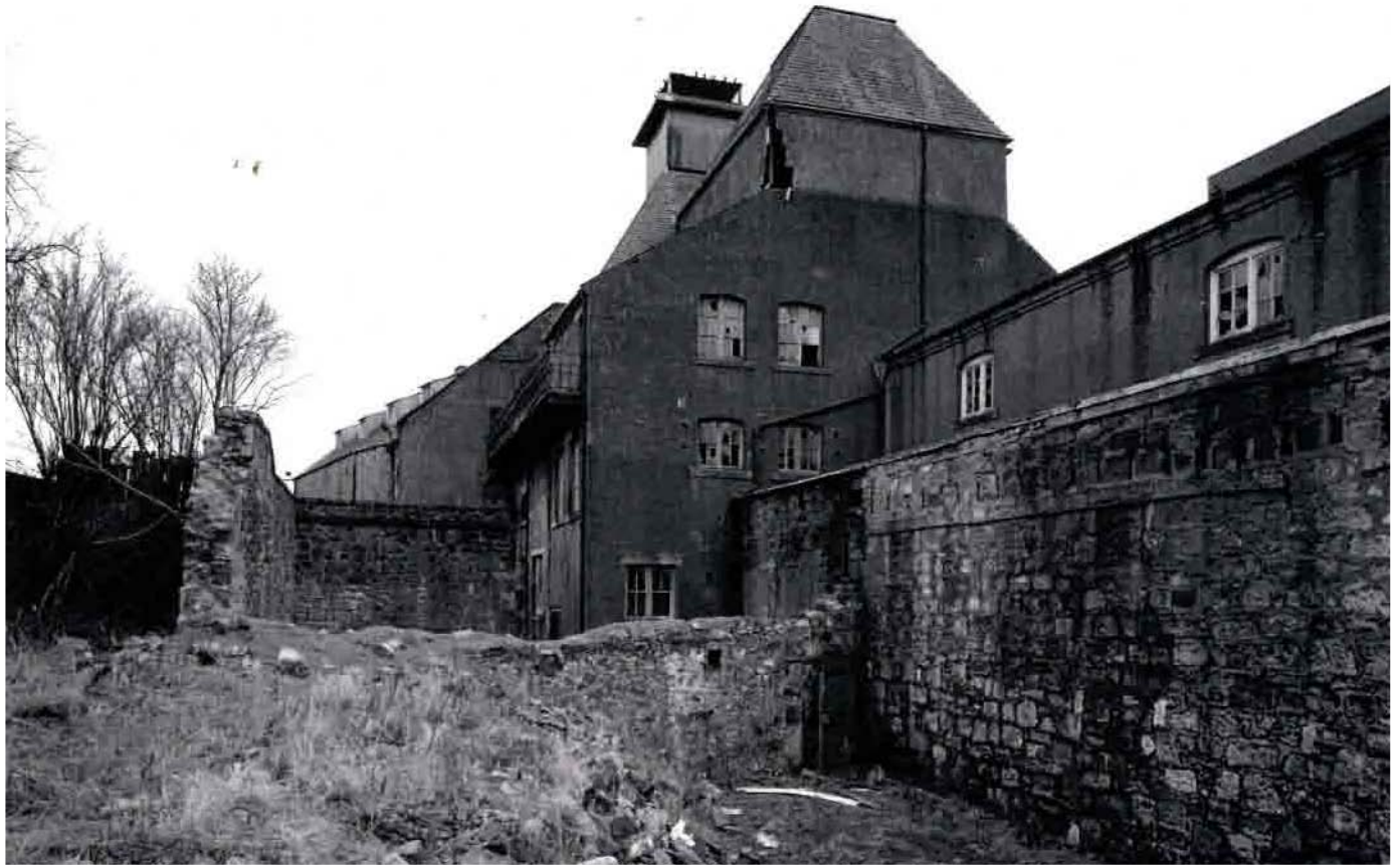
Fig. 3 - View from the southwest along south side of floor maltings attached to the west elevation of the double kiln maltings building (Source: RCAHMS, 2001, photo no. E021167)
