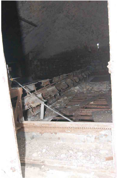
Fig. 13 - Pre-demolition shot of the rotating plough housed on the second floor
