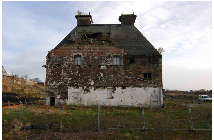
Fig. 12 - Pre-demolition shot of the west-facing elevation
