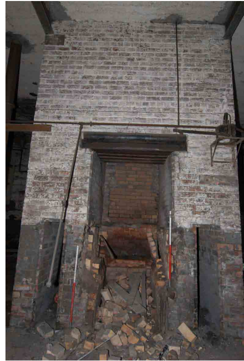
Fig. 14 - Pre-demolition shot of one of the kilns on the ground floor
