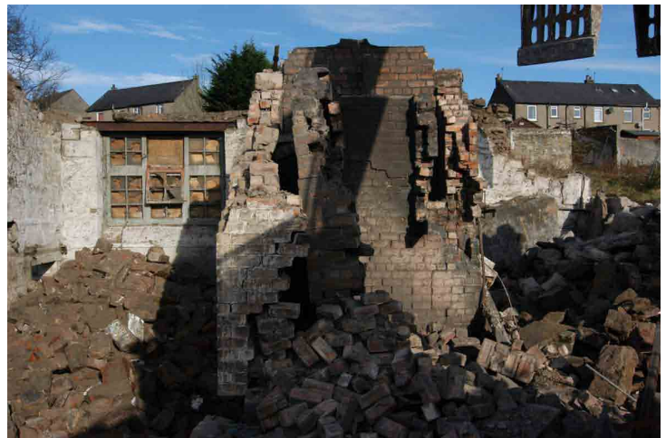
Fig. 21 - Close-up of the northern-most kiln part demolished
