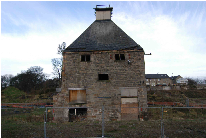
Fig. 11 - Pre-demolition shot of the south-facing elevation
