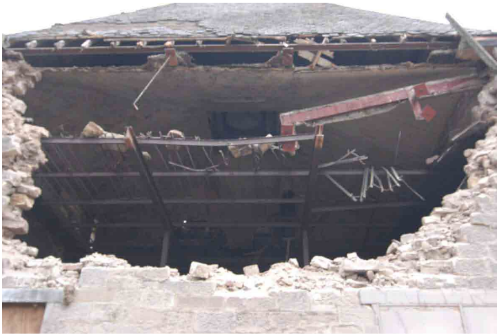
Fig. 17 - Smoke chamber exposed and structural steelwork
