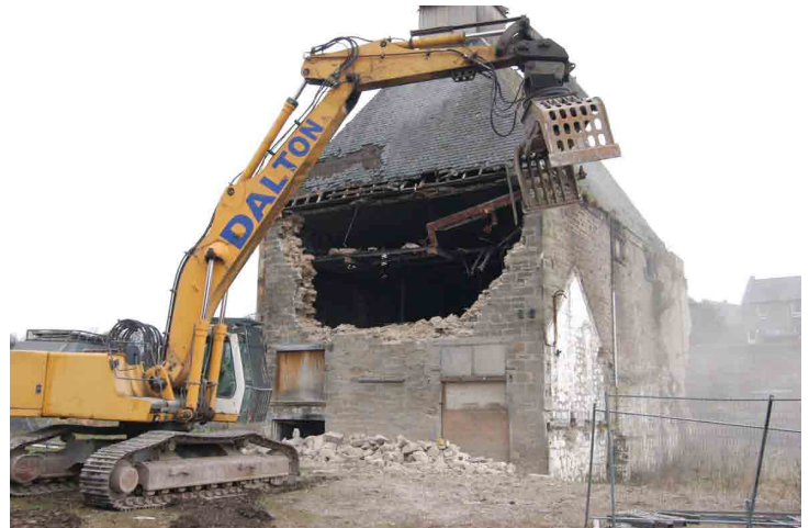
Fig. 16 - First floor steel work exposed
