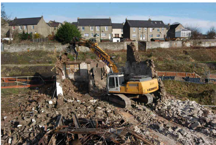
Fig. 20 - Northern-most kiln exposed within the near demolished building
