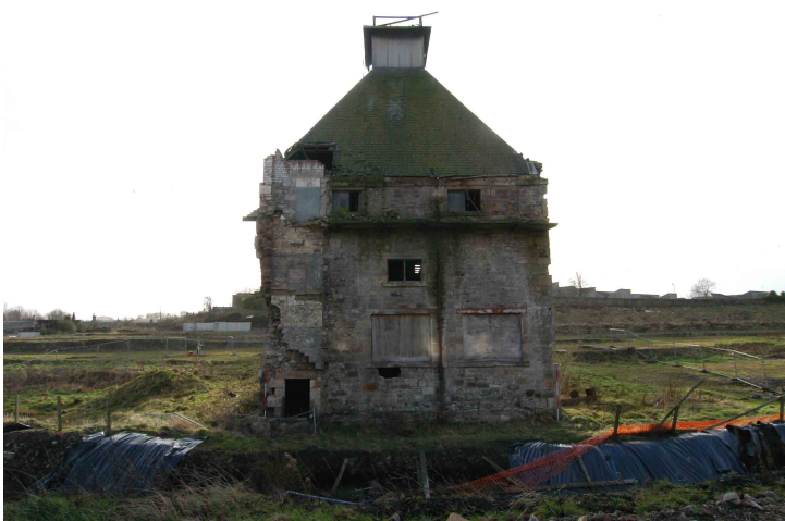
Fig. 9 - Pre-demolition shot of the north-facing elevation
