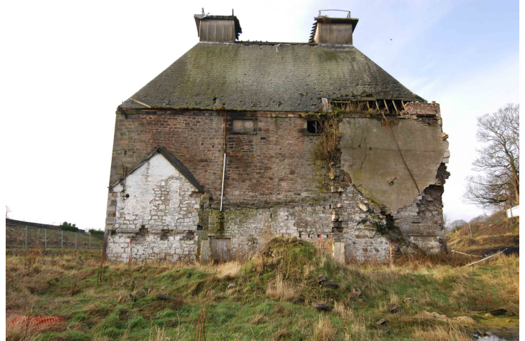
Fig. 10 - Pre-demolition shot of the east-facing elevation
