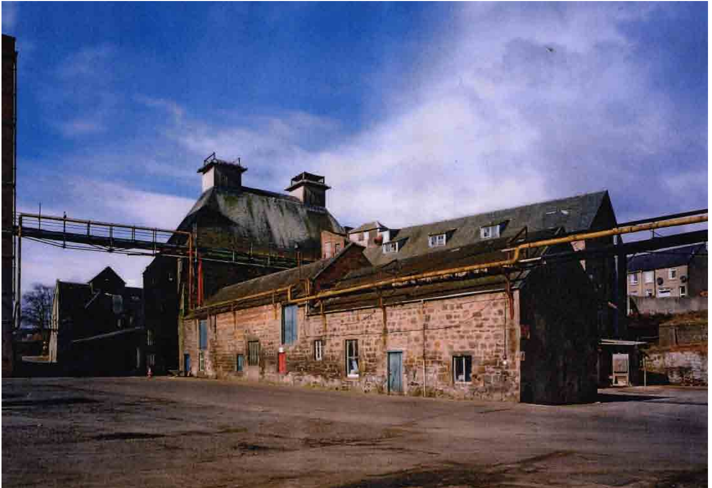
Fig. 5 - View from the east end of the old malting block with stores buildings in the foreground (Source: RCAHMS, 2001, photo no. E02145)
