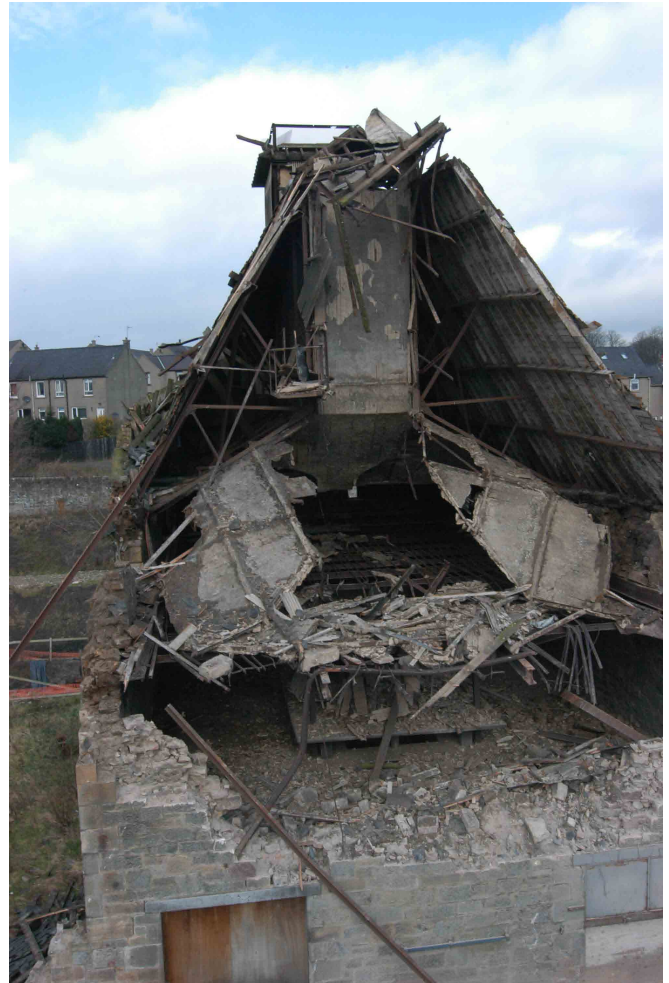
Fig. 18 - Smoke chamber and first floor baffle exposed
