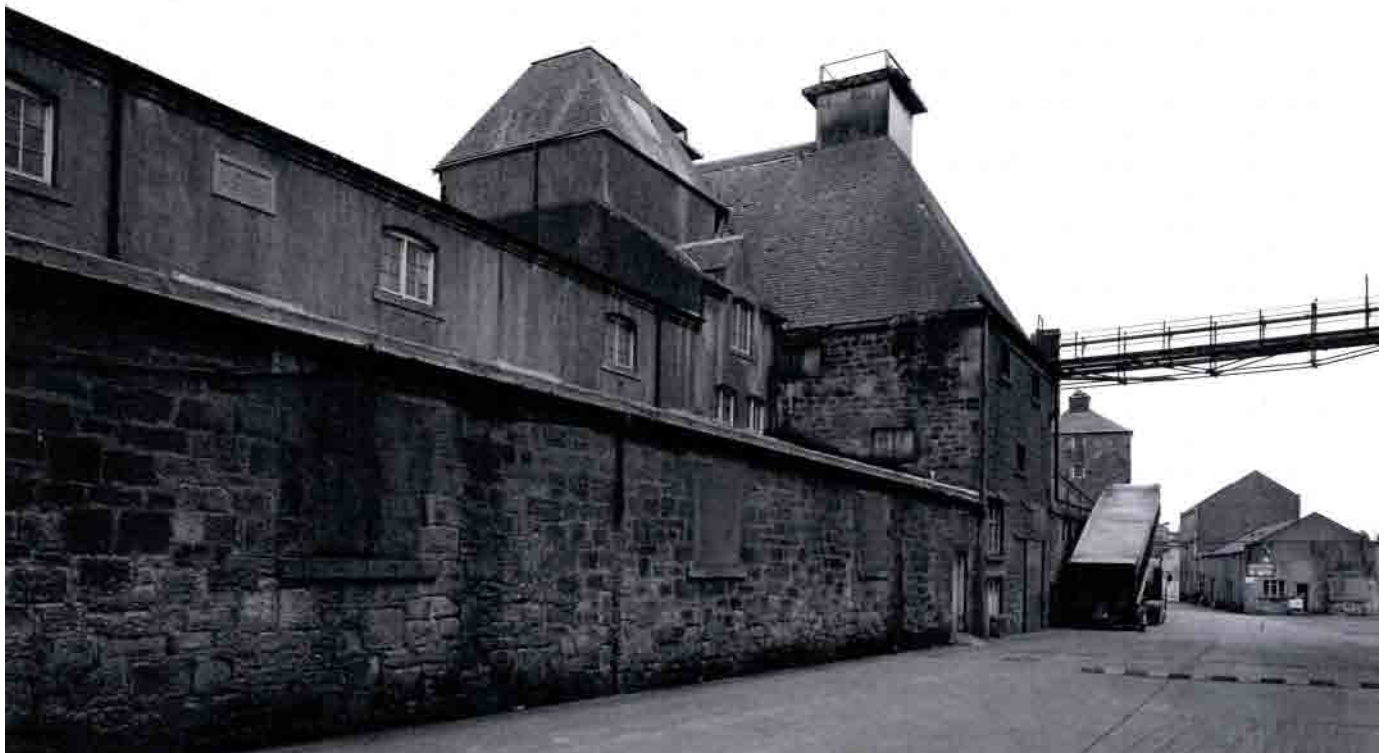
Fig. 4 - View from the northwest side of the floor malting and double kiln malting building (Source: RCAHMS, 2001, photo no. E021160)
