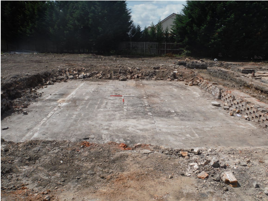
Fig. 12 - Building 1 from the east
