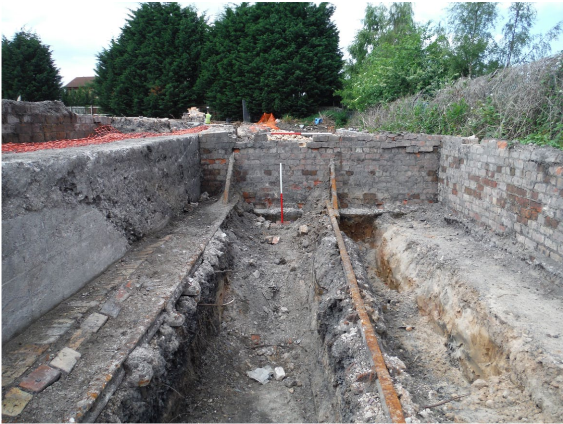
Fig. 15 - Railway Siding 1 showing wall 014
