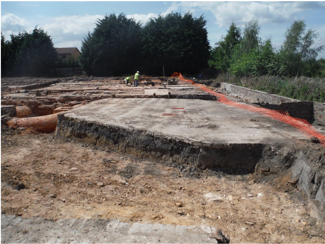
Fig. 23 - Platform 1 from east
