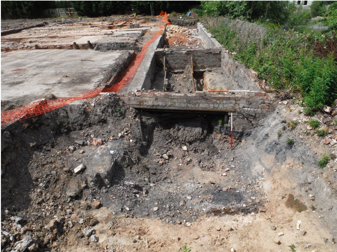
Fig. 14 - Railway Siding 1 from east
