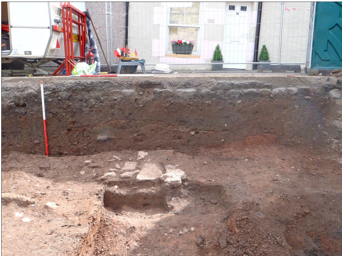
Fig. 6 - General view of site during excavation
