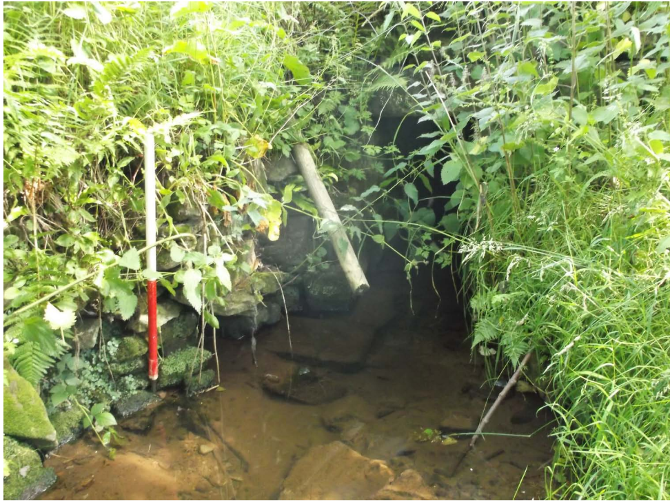
Plate 7: East culvert for burn in north of Area 6 (Site 5)
