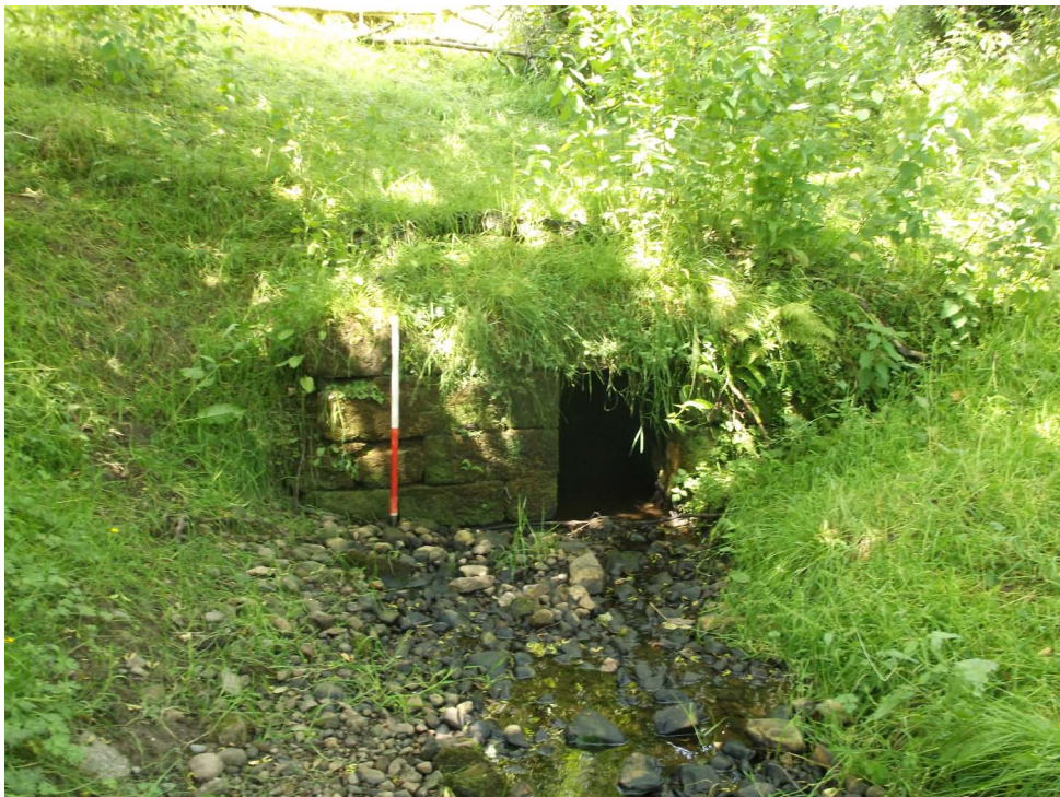
Plate 8: West culvert for burn in north of Area 6 ( Site 5)
