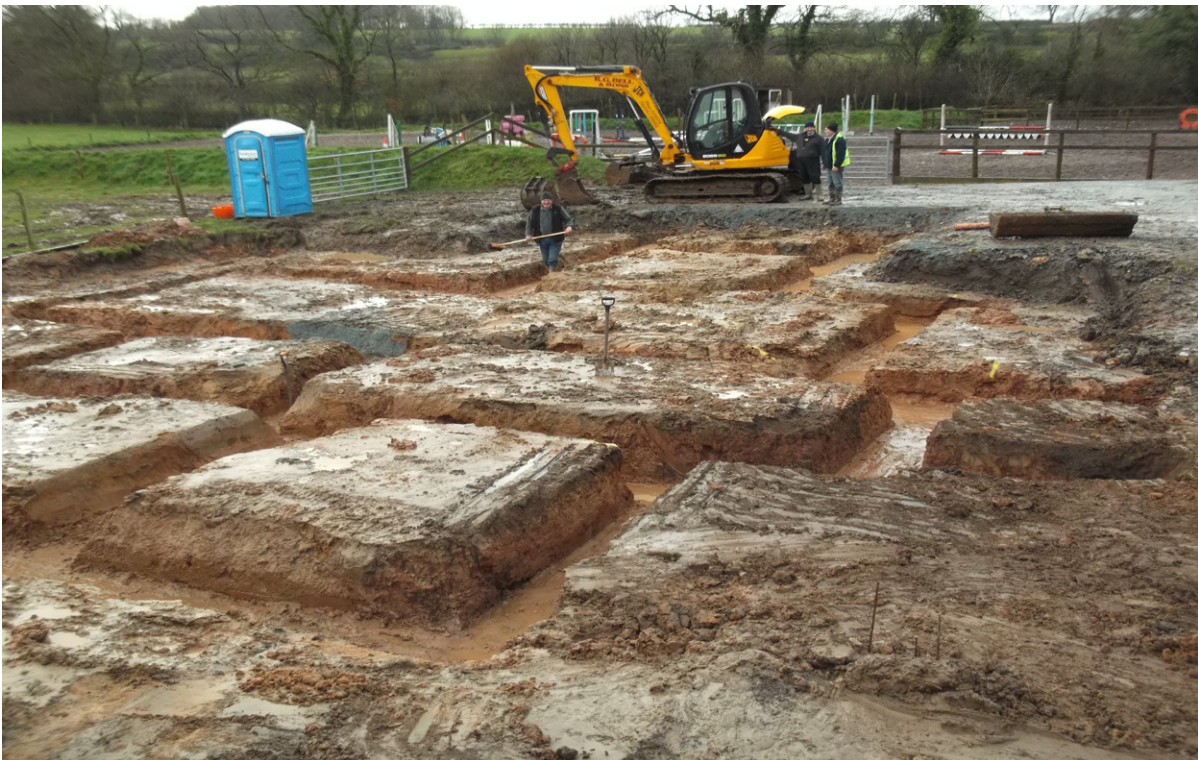
Plate 2: Site after excavation of foundation trenches, south-west facing shot
