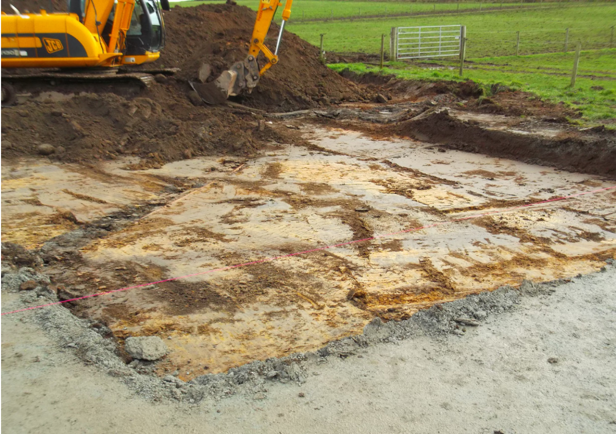
Plate 1: General site shot taken after topsoil strip, south facing shot
