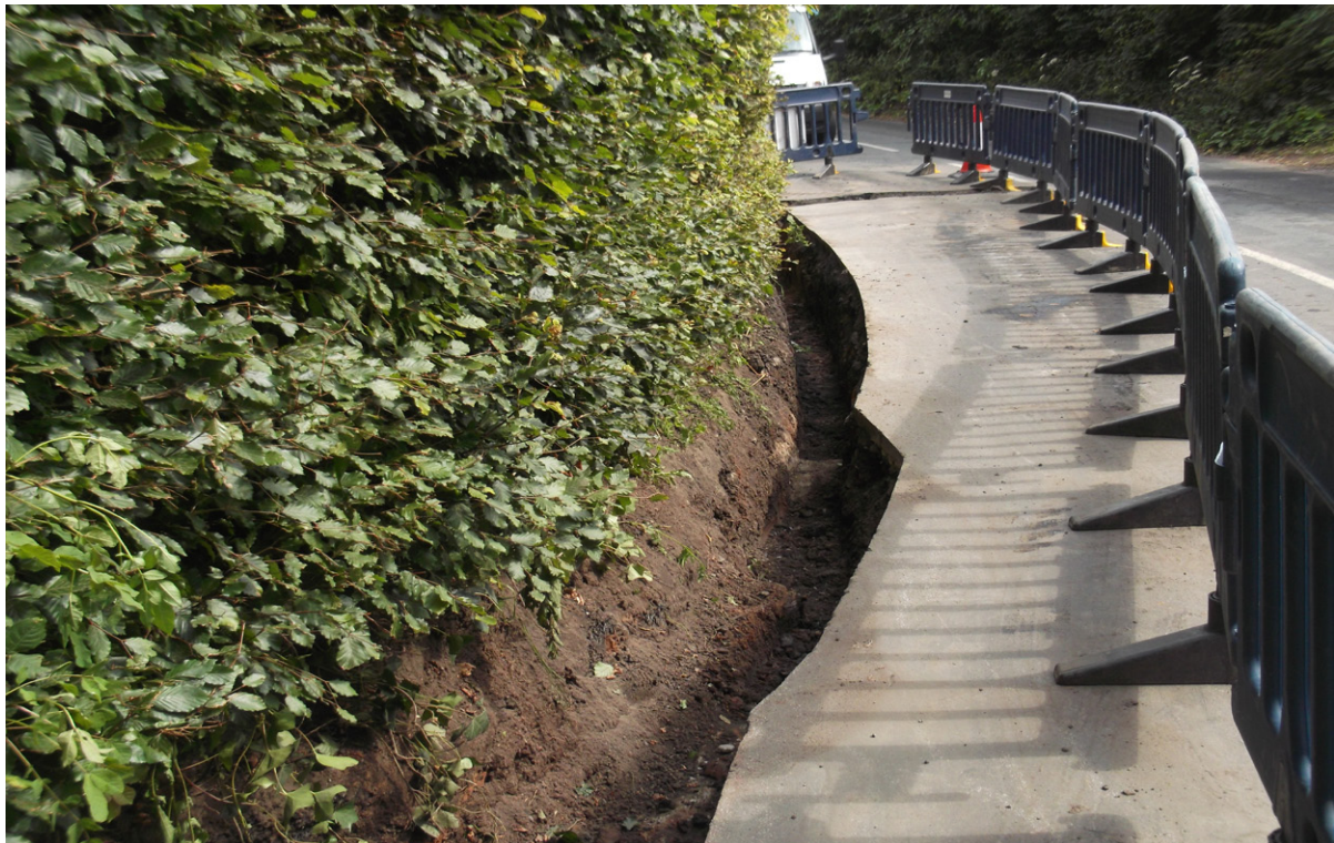
Plate 6: Service trench within existing road, looking south-east
