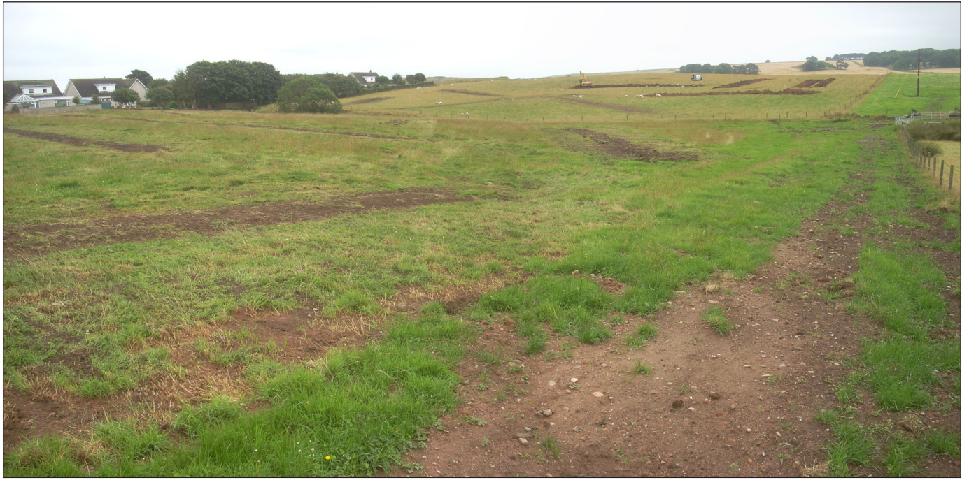
Fig. 2 - General views of the site with trenching in progress
