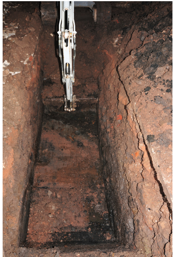
Fig. 4 - NW end of trench excavated to fullest extent
