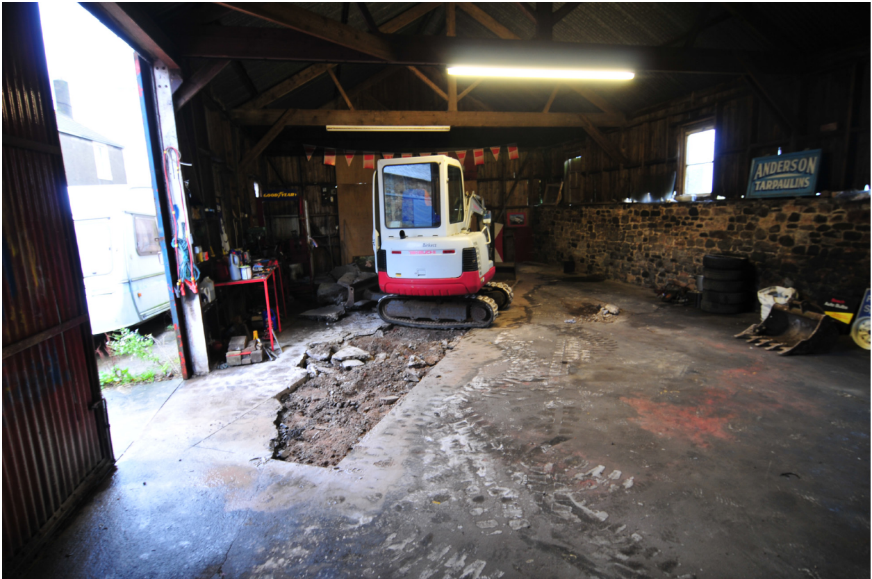
Fig. 2 - Interior of garage pre-excitation
