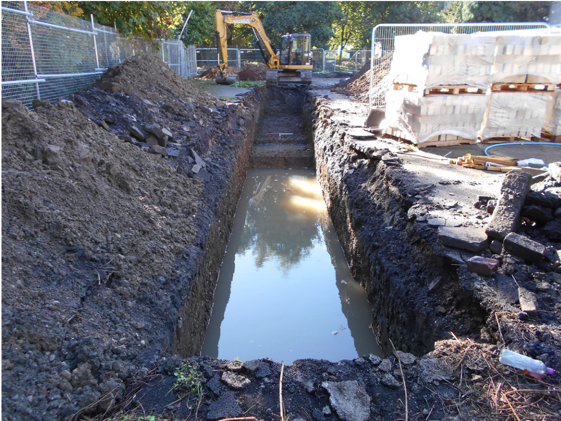
Plate 3 - View of Trench 3, facing south-south-east, showing breach in water table at north end
