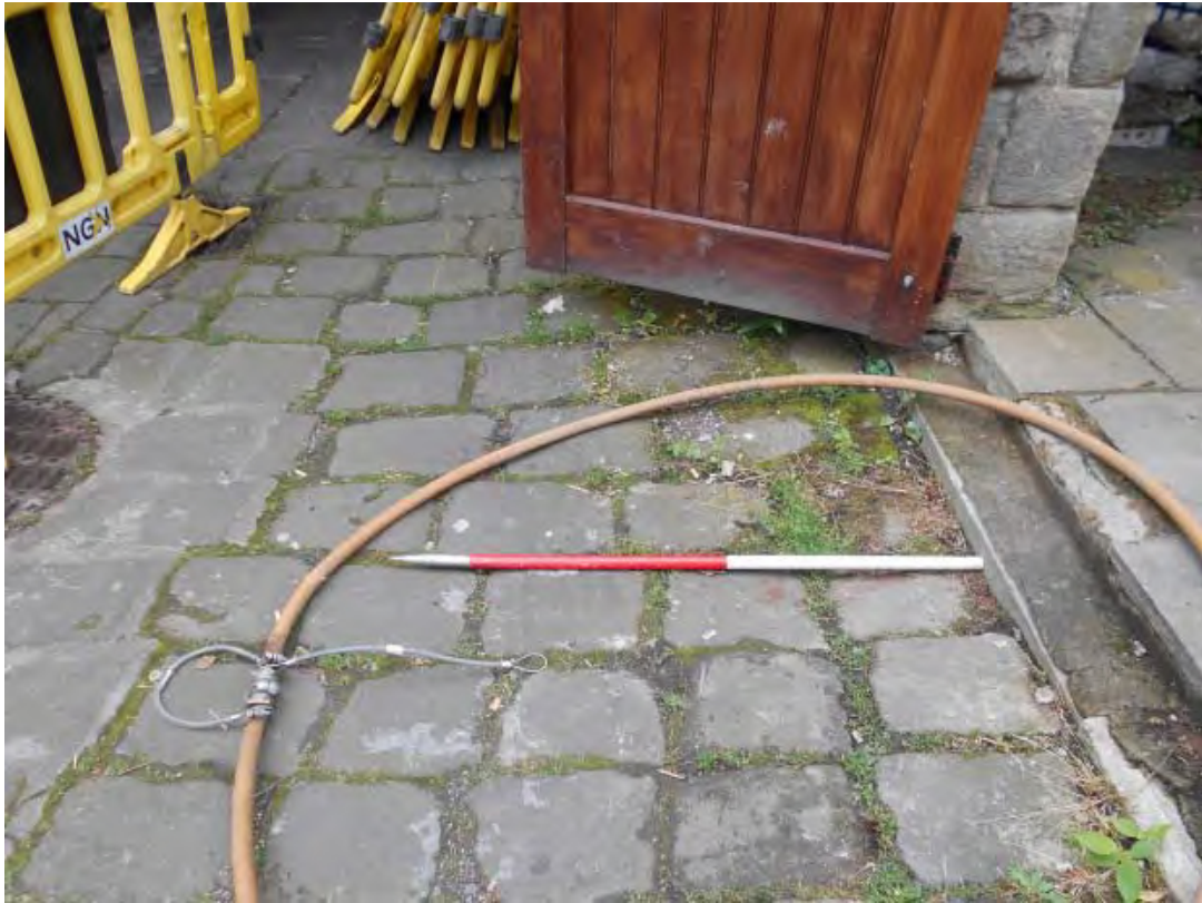
Plate 1: Pre-excavation shot of pipe trench
