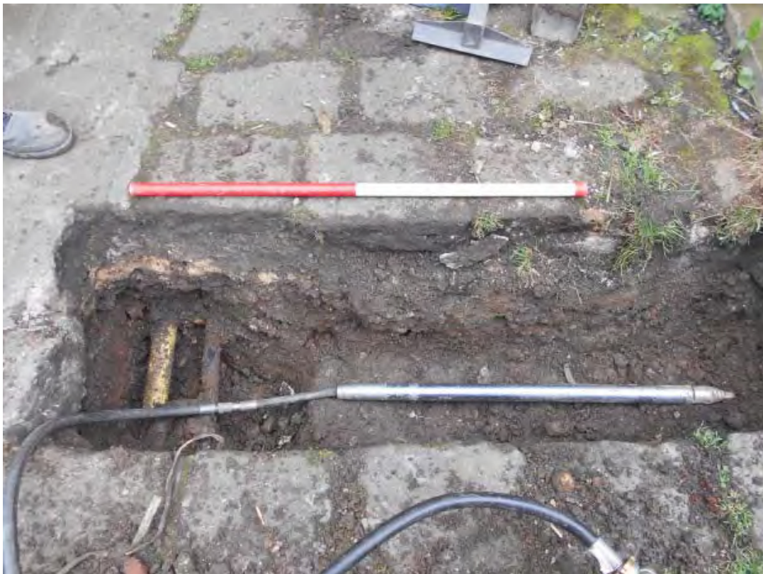
Plate 2: Post-excavation shot of pipe trench
