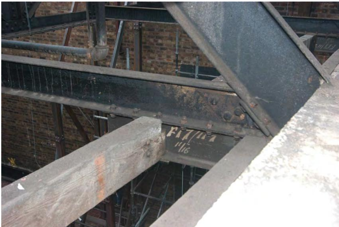
Plate 3: Cross-brace steelwork with setting out numbers and mansard jack beams (030)
