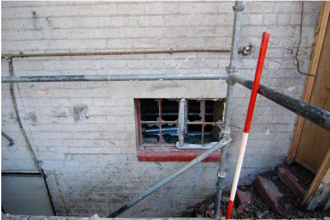
Plate 7: The external stairs and window (050)
