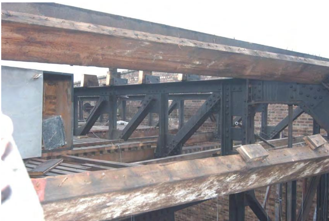
Plate 4: The transverse jack-trusses and part of the attic floor (032)
