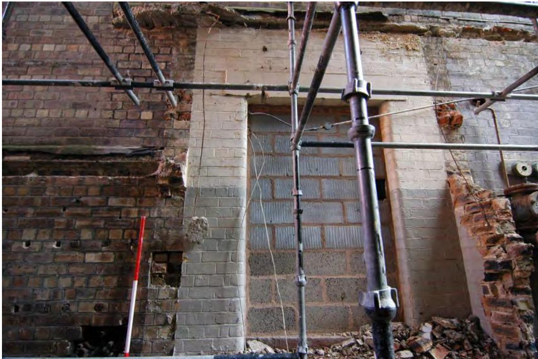
Plate 8: An external blocked entrance at the top of the demolished 1930 staircase (056)
