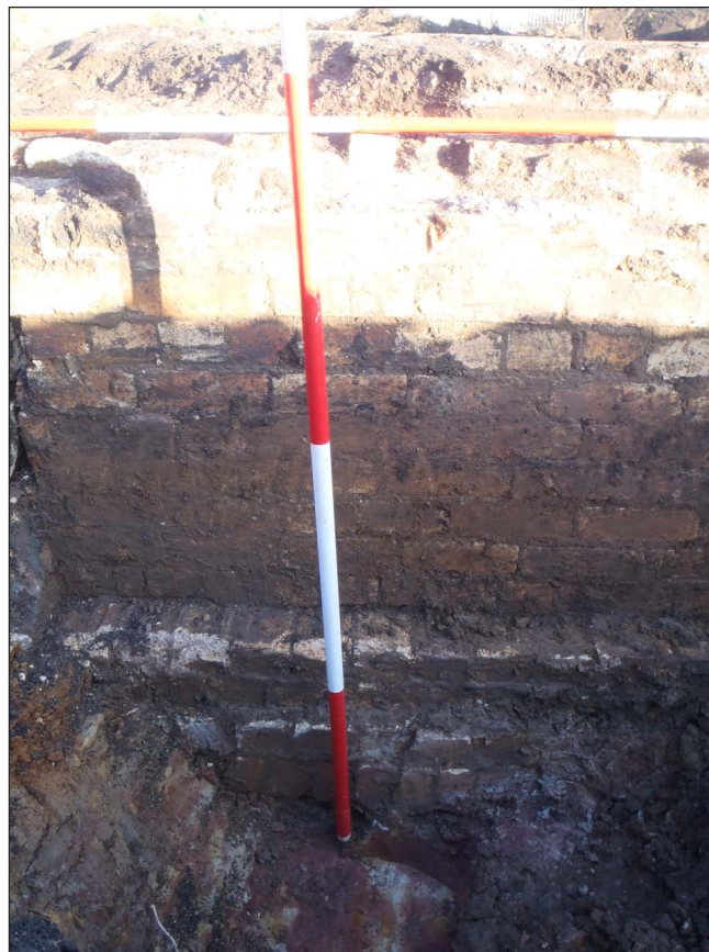
Fig. 5 – West-facing elevation of wall 003 showing foundation footing
