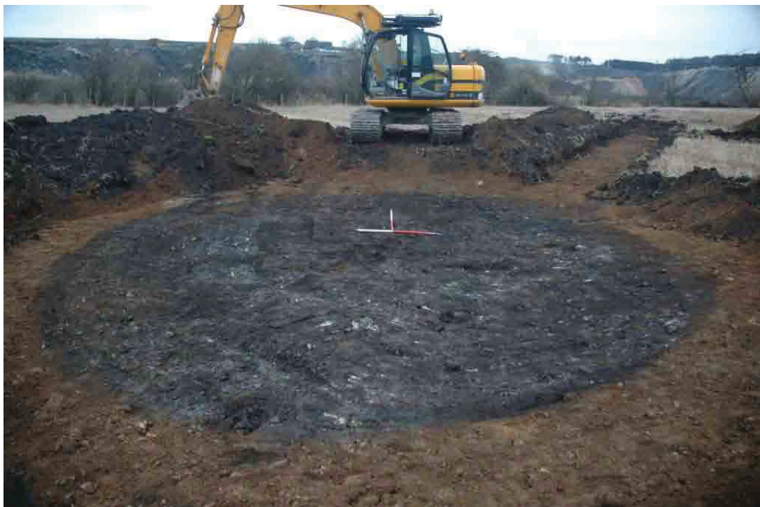
Fig. 6 - Back-filled mine-shaft
