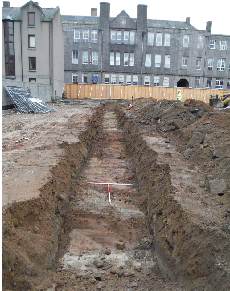
Fig. 6 - Trench 4 from the Northwest
