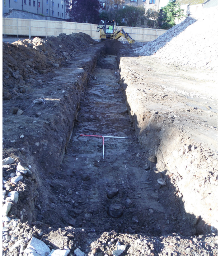
Fig. 3 - Trench 2 from the Southeast
