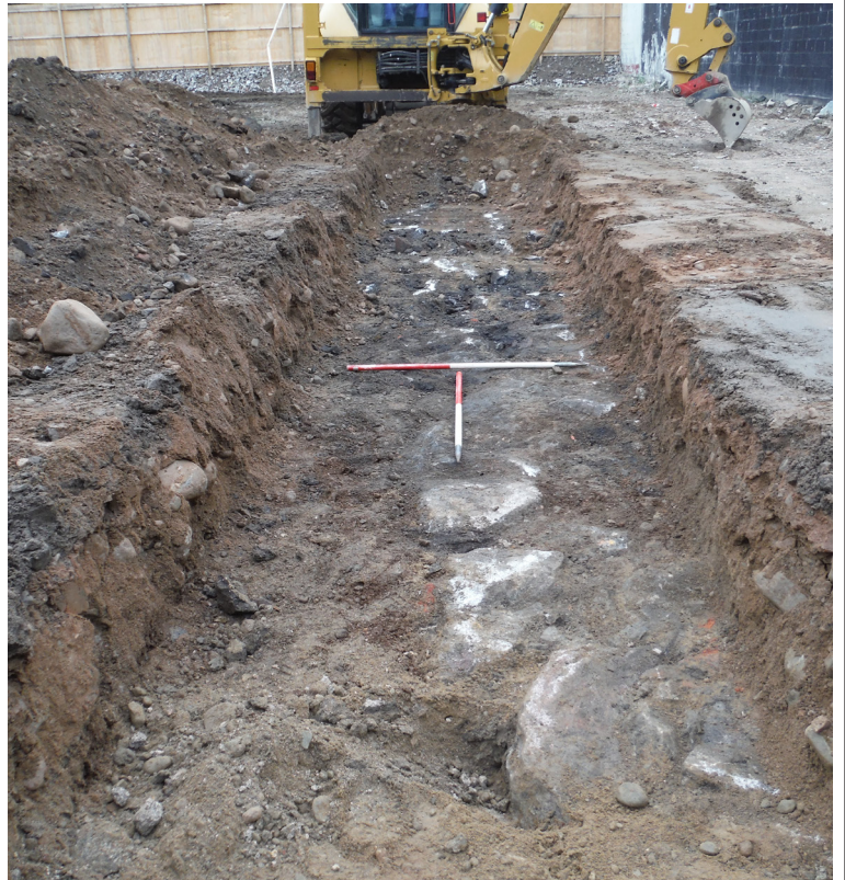
Fig. 5 - Trench 4 from Southeast showing demolition/levelling deposit 004
