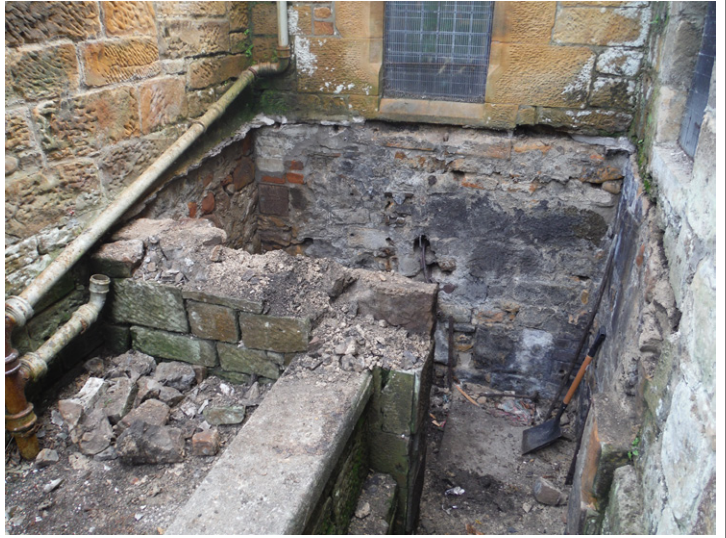
Fig. 3 - External boiler house demolished.
