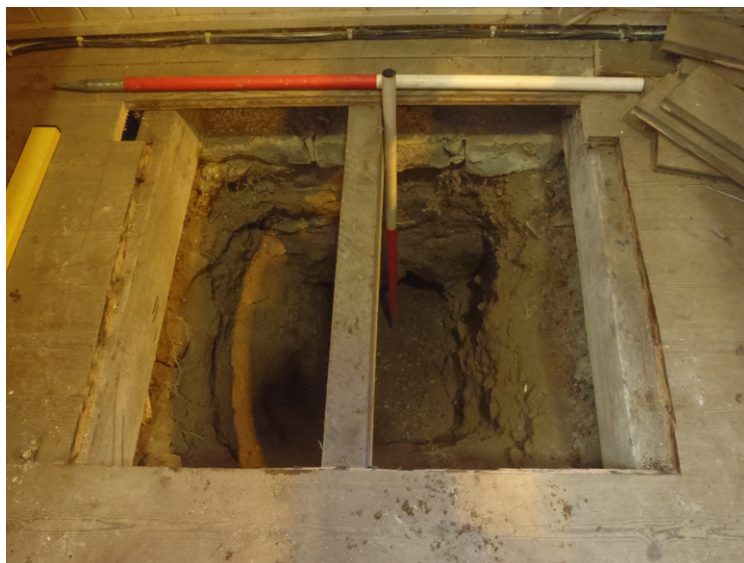
Fig. 14 - Service connection hole excavated.
