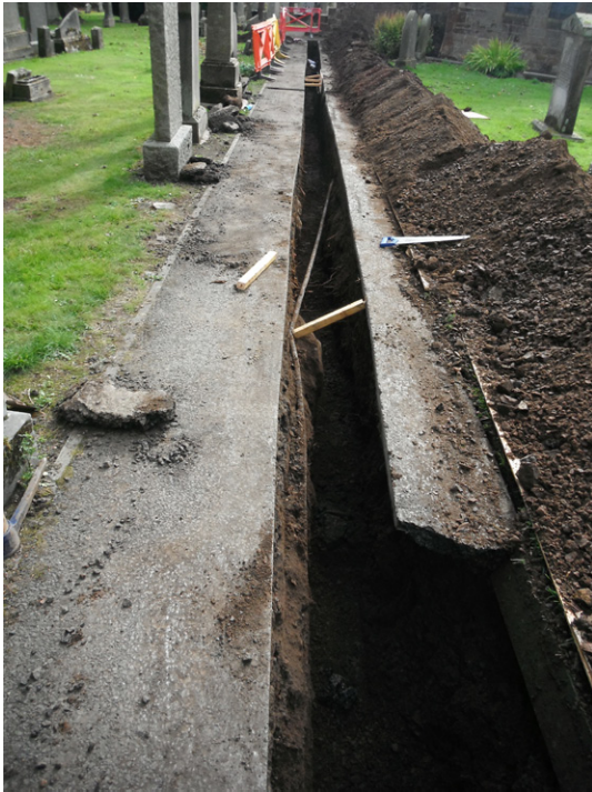
Fig. 8 - Church path excavated to follow the route of existing service trench.
