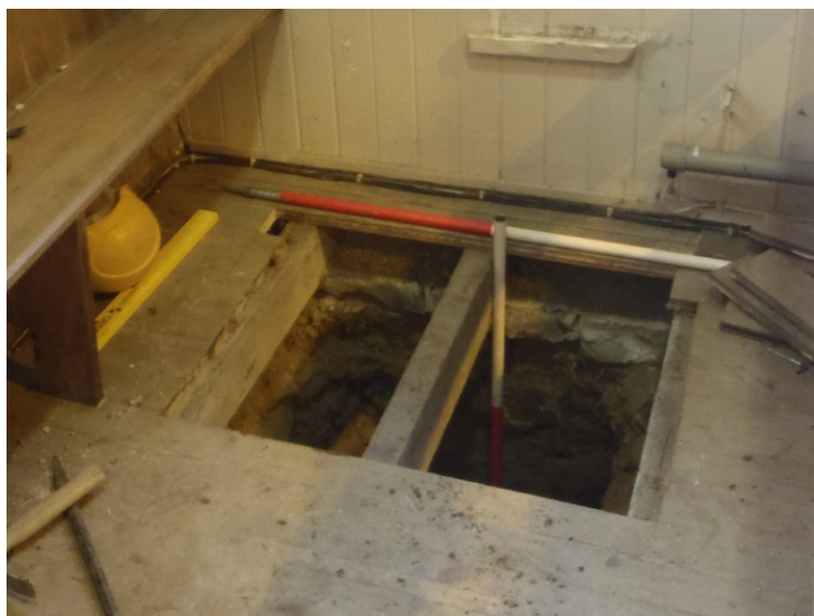
Fig. 13 - Service connection hole dug into the aisle floor.
