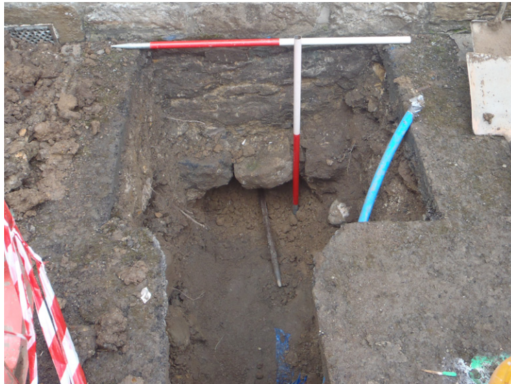
Fig. 12 - Manhole dug to formation level showing foundation course of the church.
