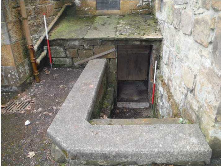
Fig. 2 - External boiler house prior to demolition.
