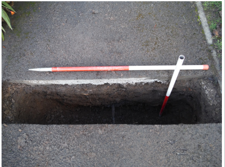
Fig. 7 - One of three test pits dug into the church yard path.
