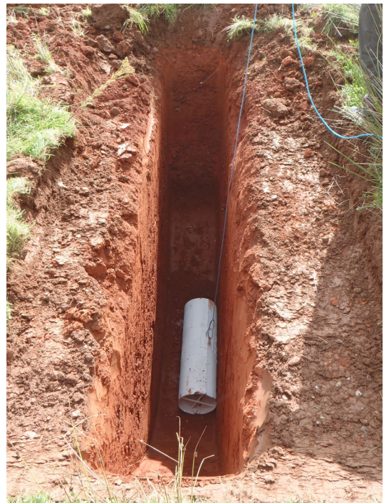
Fig 5 - Test-pit fully excavated.
