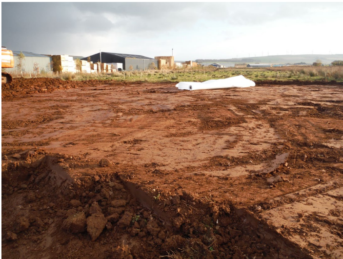
Fig. 4 - Crane pad/hardstanding excavated to formation level.
