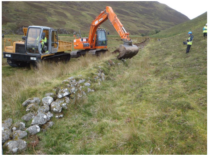
Fig. 10 - Removal of wall A2.
