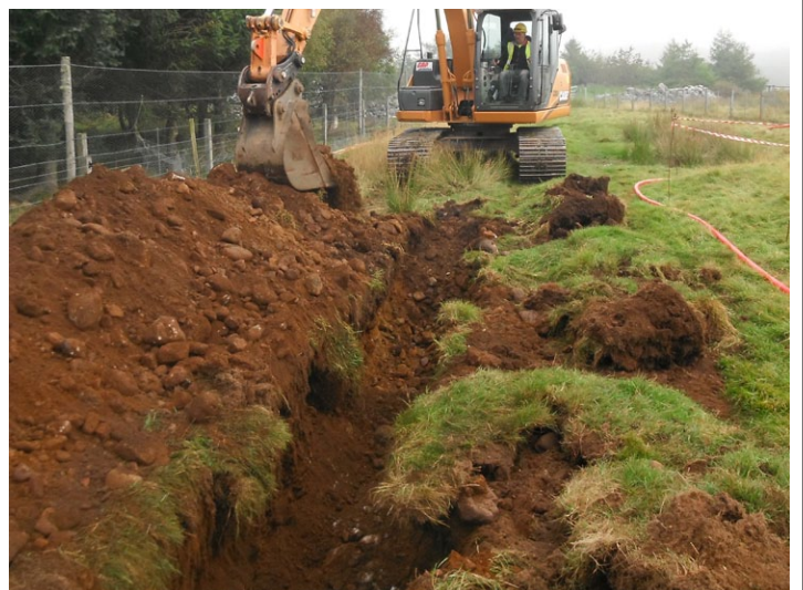
Fig. 20 - Cable trench alongside demarcated feature in Fig 18.
