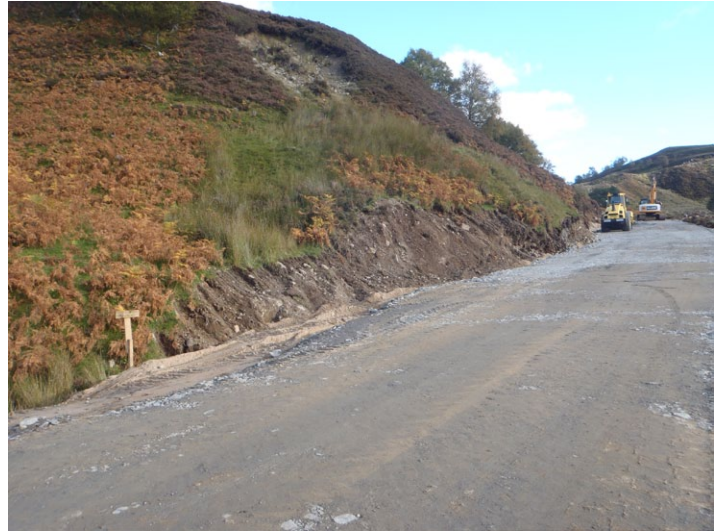
Fig. 6 - General shot of road works on haul road.
