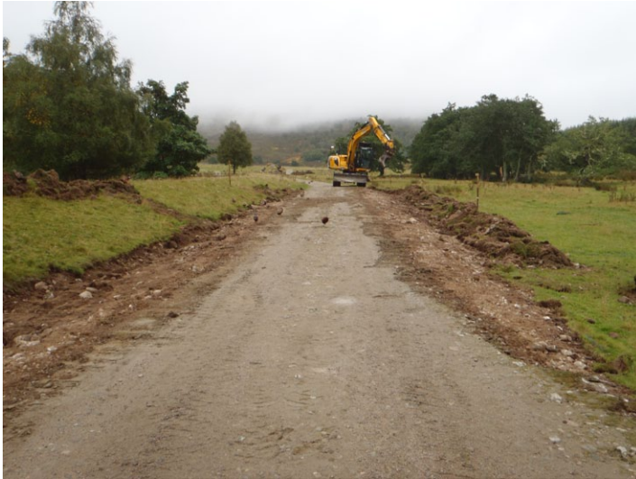
Fig. 5 - General shot of road works on haul road.
