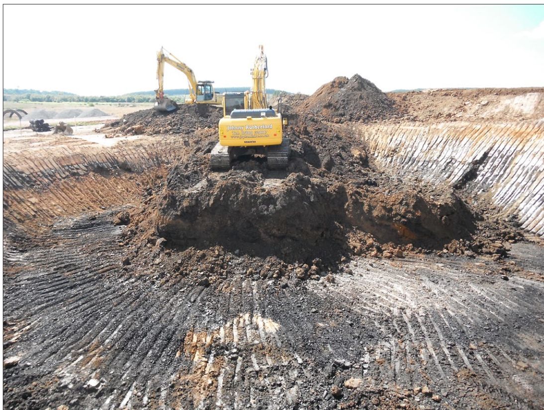
Fig. 10 - Deep working by a mechanical excavator exposing near surface coal and shale deposits
