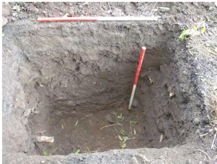
Fig. 5: BH1, south-facing section
