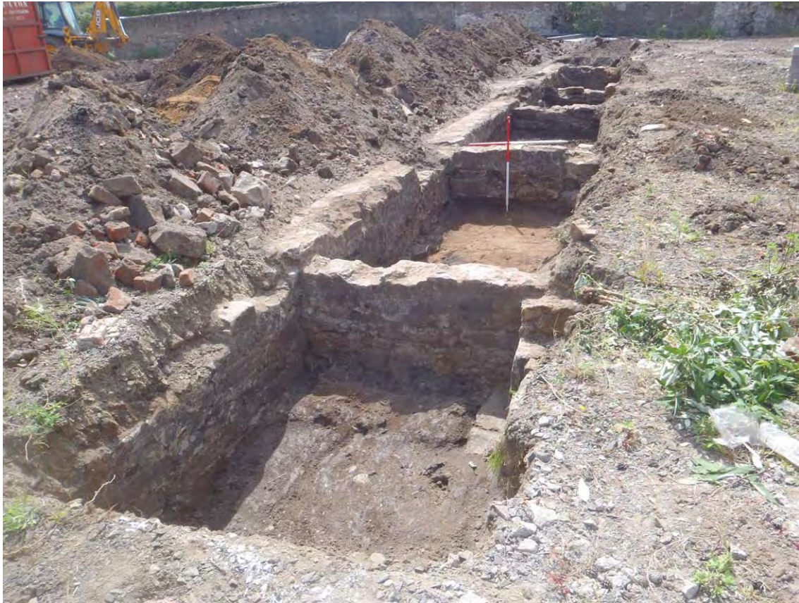
Fig. 7. - Trench1 wall footings from the north
