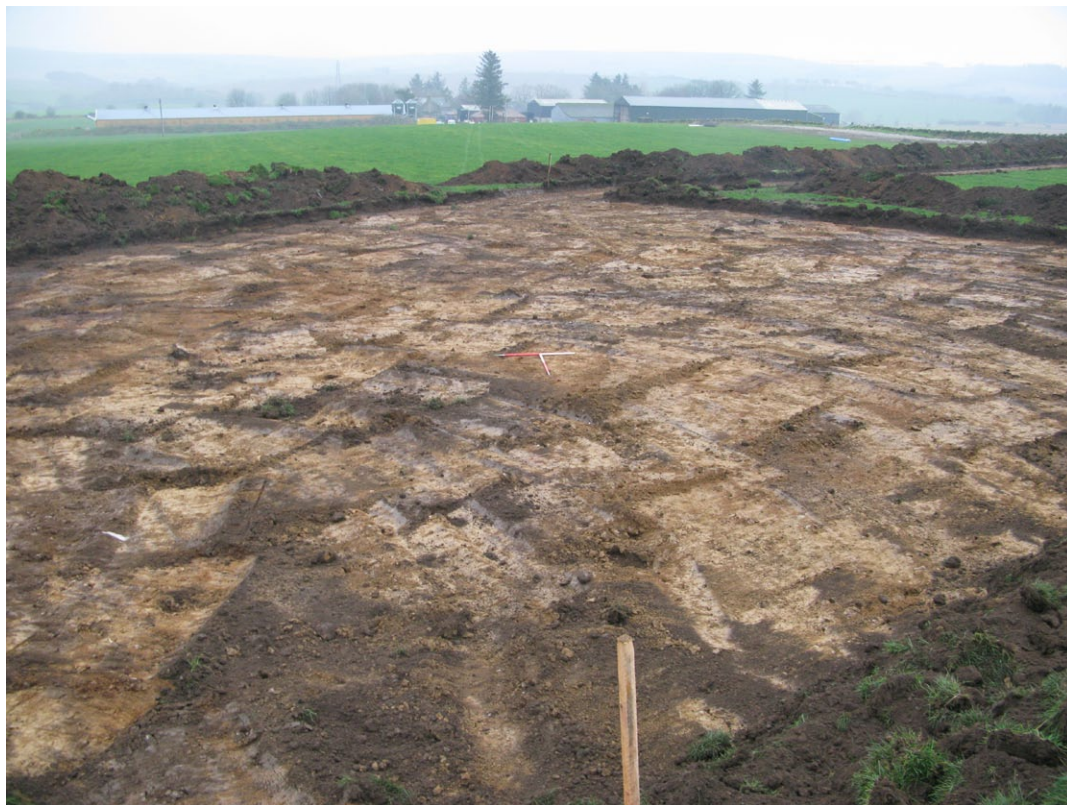
Fig. 3 - Turbine base and hard standing area
