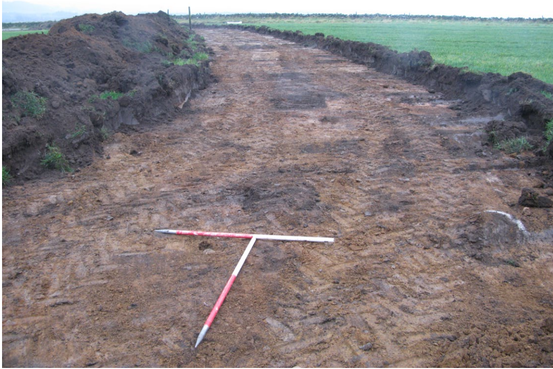
Fig. 2 - Access track to turbine
