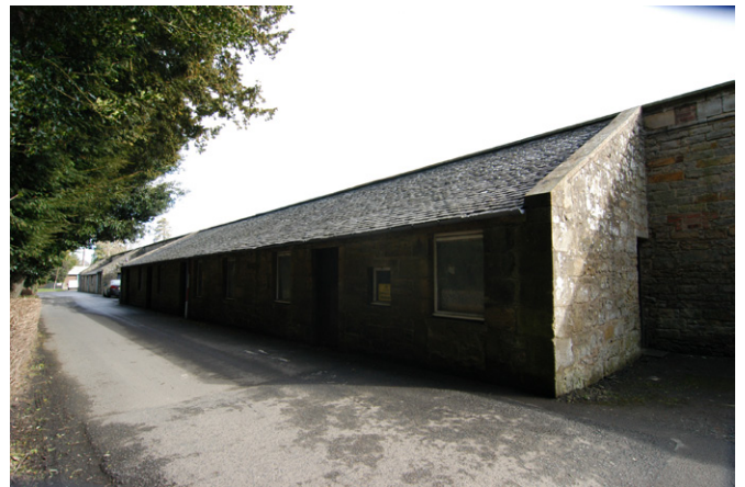
Plate 12 - Exterior NW-facing elevation, Building B
