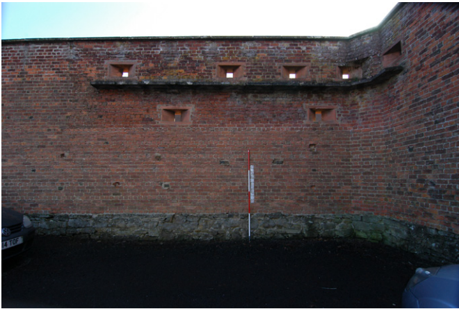
Plate 3 - Interior NW-facing elevation, west corner with splayed openings
