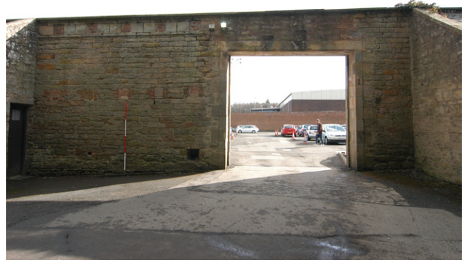
Plate 14 - Exterior NW-facing elevation, main vehicular access into the walled garden with blocked hatch vents on its left hand side
