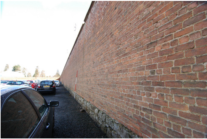
Plate 1 - Interior NW-facing elevation, general oblique view
