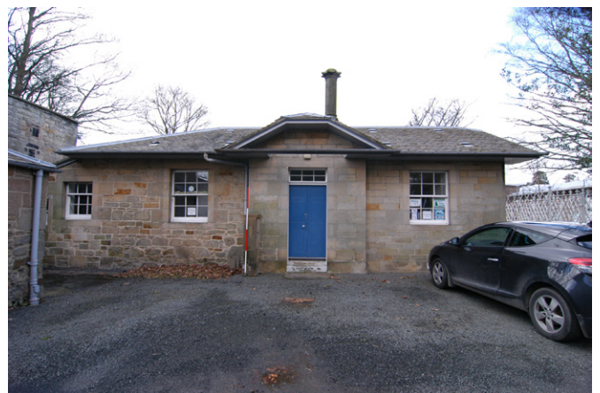
Plate 16 - NE-facing elevation of Building D (Gardener's Cottage) built against the walled garden
