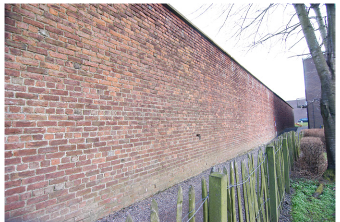
Plate 18 - Exterior SW-facing elevation, general view
