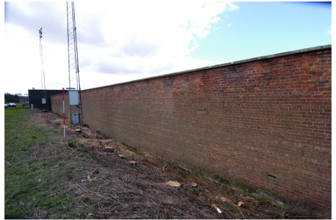
Plate 10 - Exterior SE-facing elevation, general view
