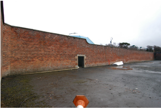
Plate 9 - Interior SW-facing elevation, general view
