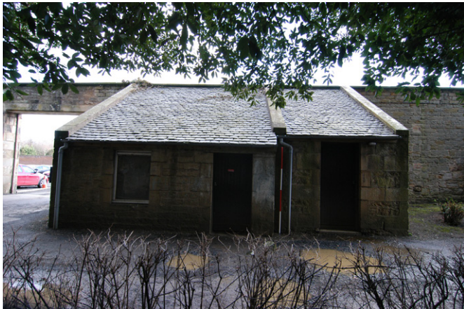
Plate 15 - Exterior NW-facing elevation, Building C
