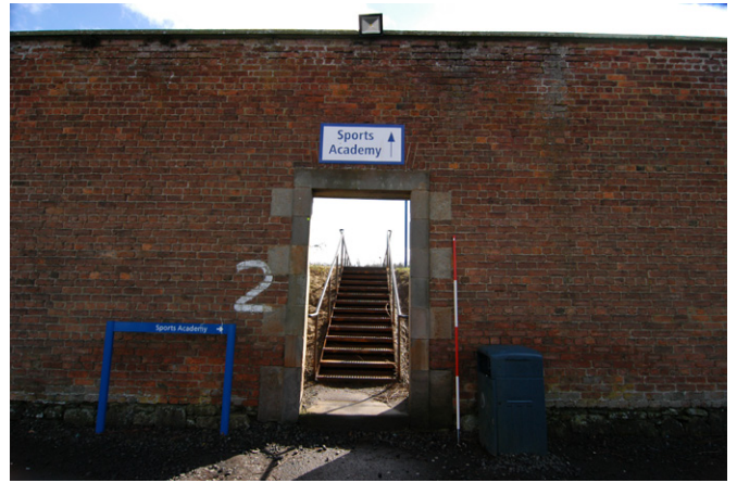
Plate 2 - Interior NW-facing elevation, central doorway
