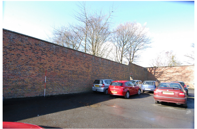
Plate 4 - Interior NE-facing elevation, general view
