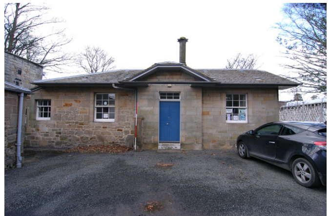
Plate 16 - NE-facing elevation of Building D (Gardener's Cottage) built against the walled garden
