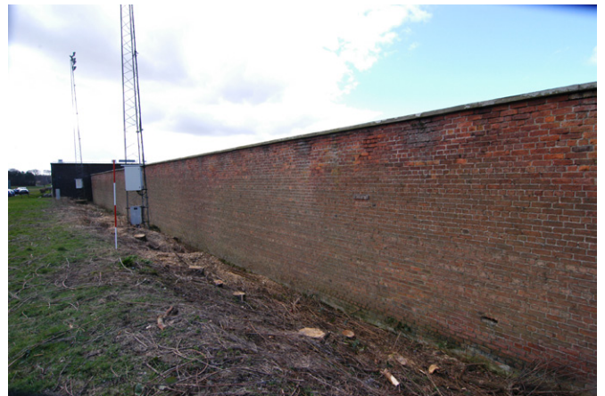
Plate 10 - Exterior SE-facing elevation, general view
