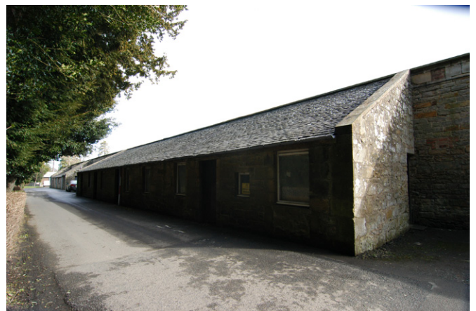
Plate 12 - Exterior NW-facing elevation, Building B
