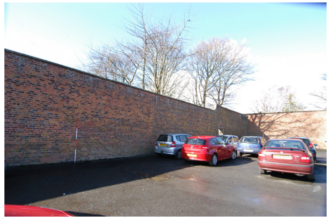
Plate 4 - Interior NE-facing elevation, general view
