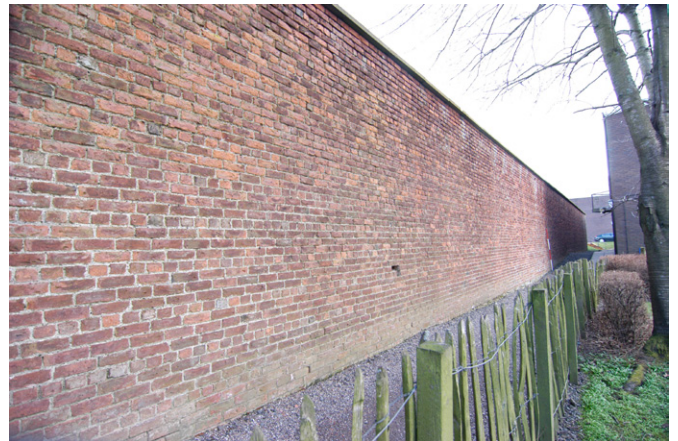
Plate 18 - Exterior SW-facing elevation, general view
