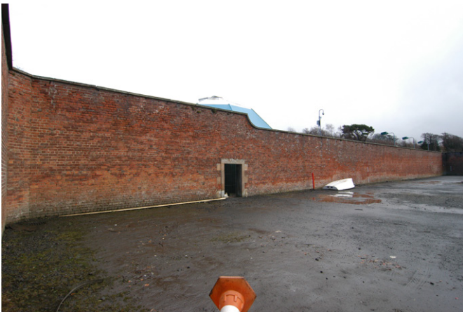
Plate 9 - Interior SW-facing elevation, general view
