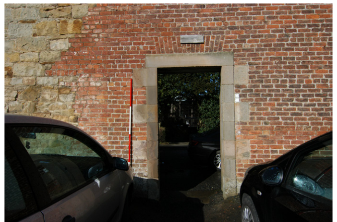
Plate 6 - Interior SE-facing elevation, doorway and the junction between brick and stonework
