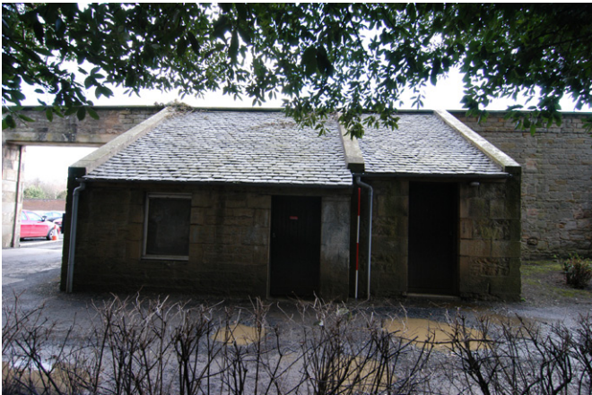
Plate 15 - Exterior NW-facing elevation, Building C
