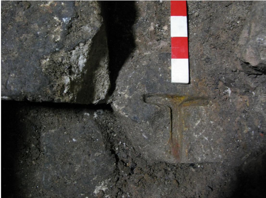
Fig. 10 - 'T'-shaped socket in foundation course **508**
