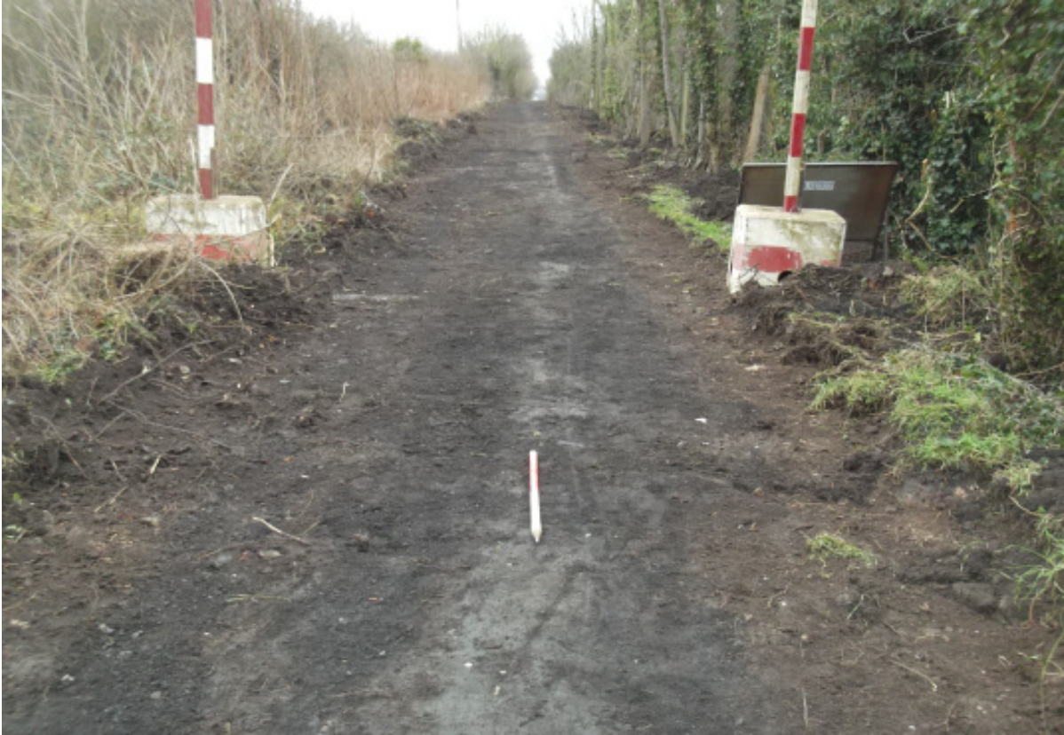
Fig. 2 - Shot of stripped cycle path looking towards A638
