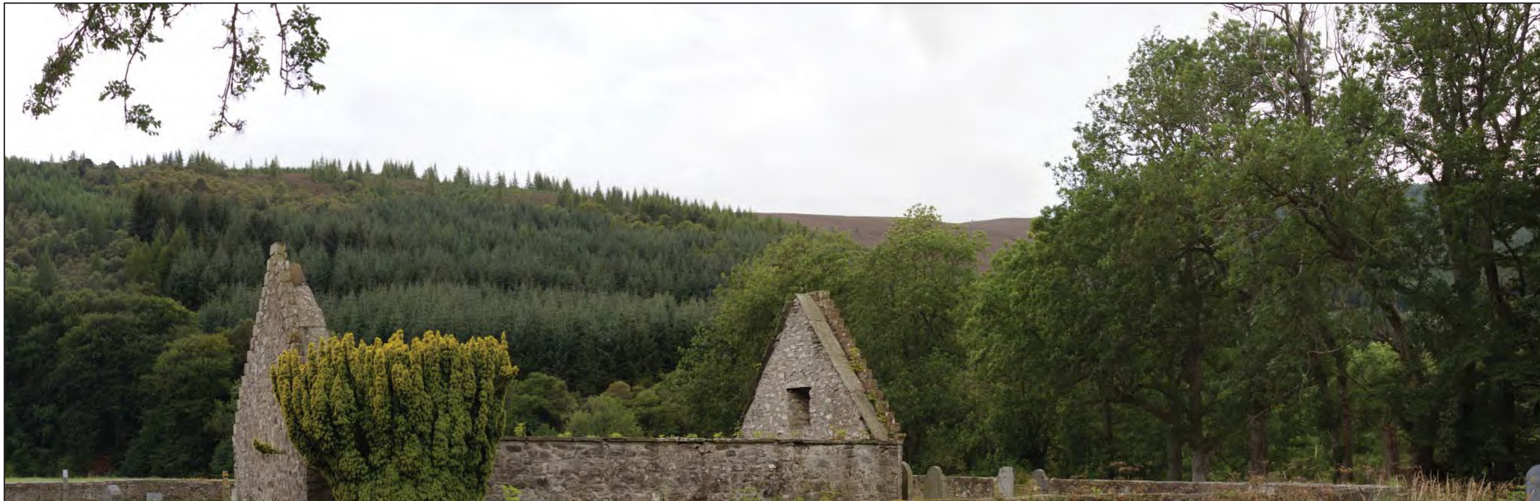
Existing view. Forbes Church and Burial Ground Scheduled Monument (Index No 11011). View of church from north-north-east. (72 degrees horizontal field of view, 32 cm viewing distance)
