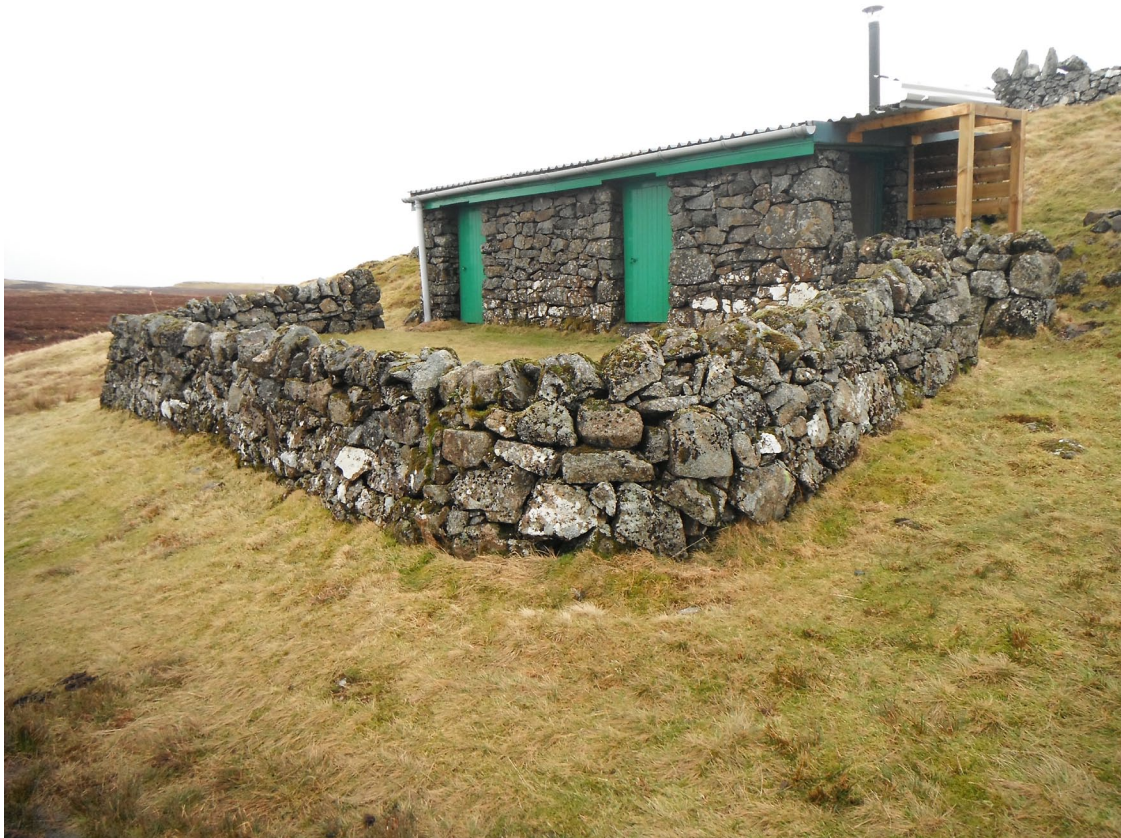
Fig. 4 Site 3, a bothy, adjacent to the existing track
