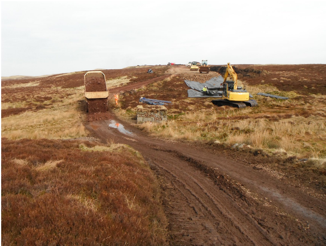
Fig. 6 The new access road passing to the east of Site 2
