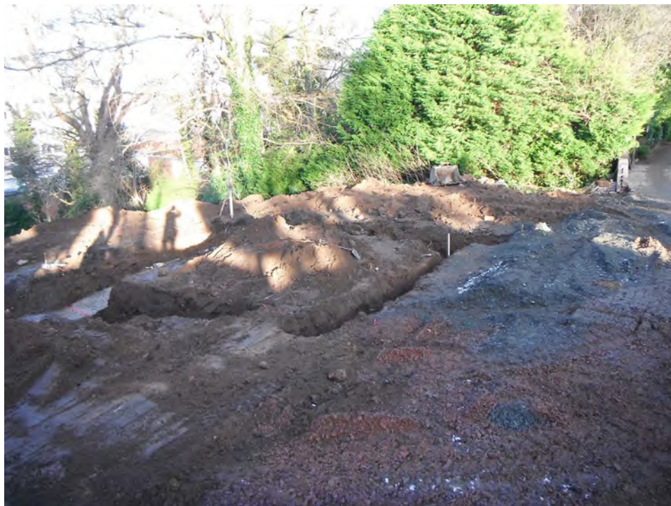
Fig. 5 - Site following foundation excavation
