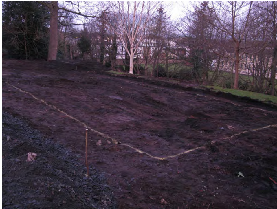
Fig. 2 - Site prior to foundation excavation
