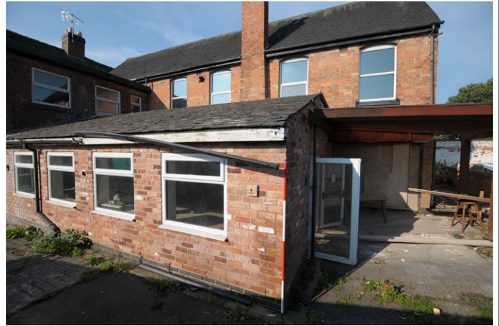
Fig. 47 - The exterior of Unit 5, looking south-west
