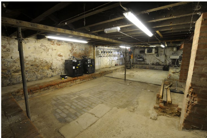
Fig. 9 - The Cellar, Unit 1, looking north-east
