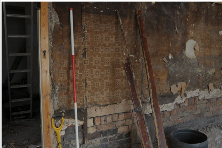
Fig. 15 - Shot of blocked doorway in north wall, ground floor, Unit 1, looking north
