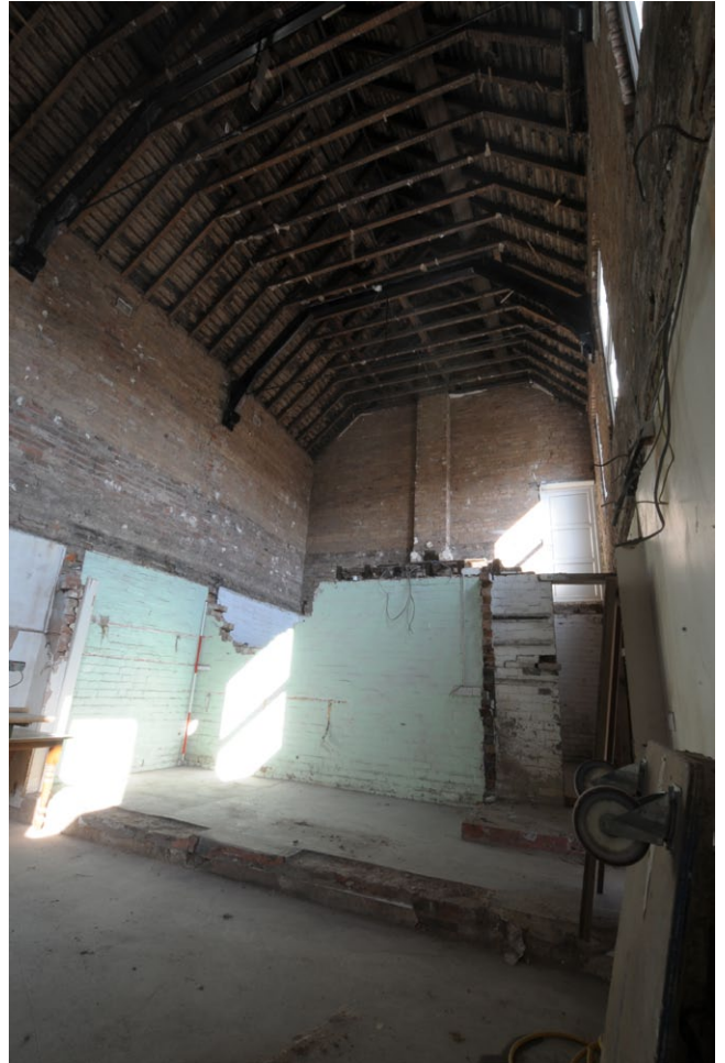
Fig. 43 - Internal view of Unit 4 after ceiling removed, looking south-east
