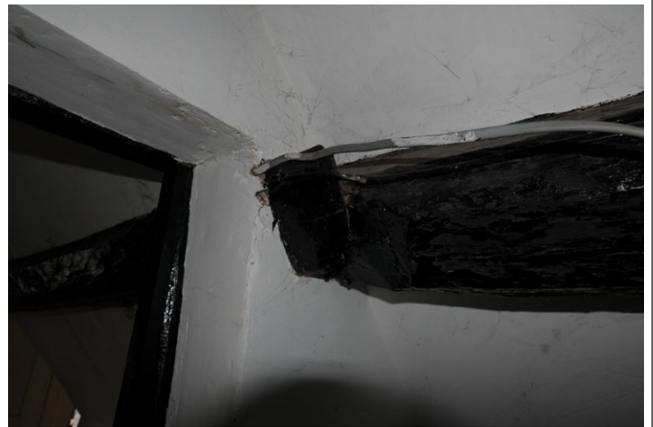
Fig. 34 - Splayed scarf joint for hewn purlins on north pitch of roof, 2nd floor (attic), Unit 1, looking north-west
