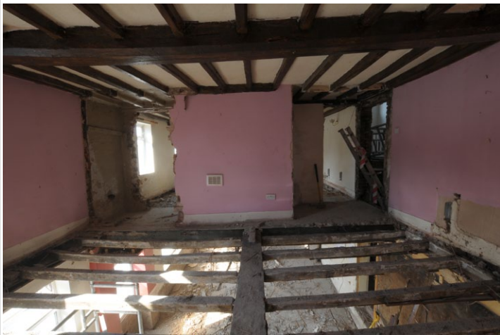
Fig. 21 - Shot of east room, 1st floor, Unit 1, looking west
