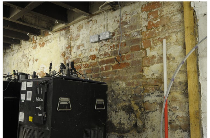
Fig. 49 - Original bricks above stone foundations, Cellar, Unit 1, looking north-west. Patching of walls in later brick can be seen on either side
