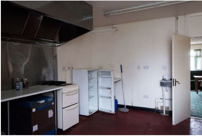
Fig. 42 - Lower floor of Unit 4, looking east
