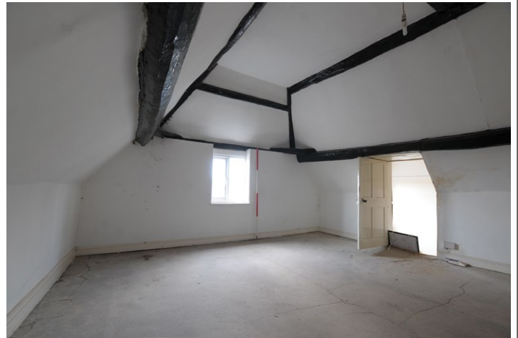
Fig. 28 - The west room, 2nd floor (attic), Unit 1, looking north-west
