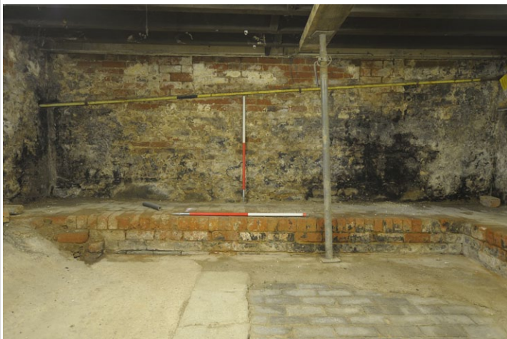
Fig. 11 - West elevation of Cellar, Unit 1, looking west
