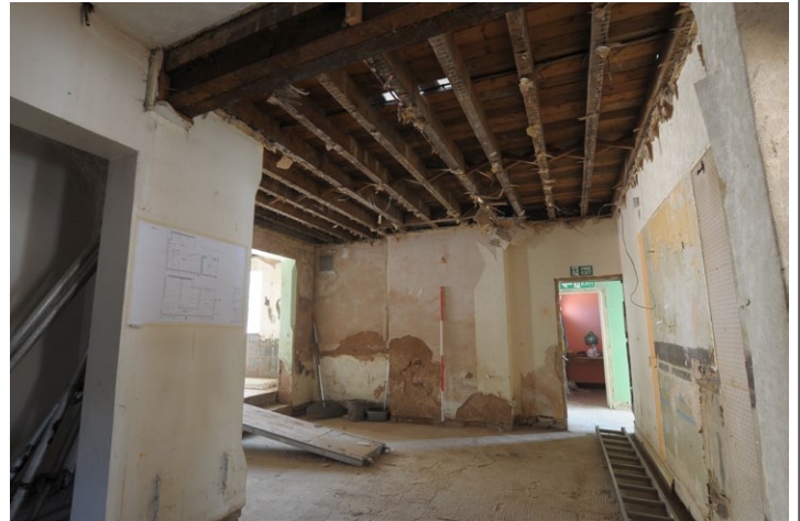
Fig. 39 - Internal view of lower floor of Unit 3 after ceiling and walls stripped, looking east
