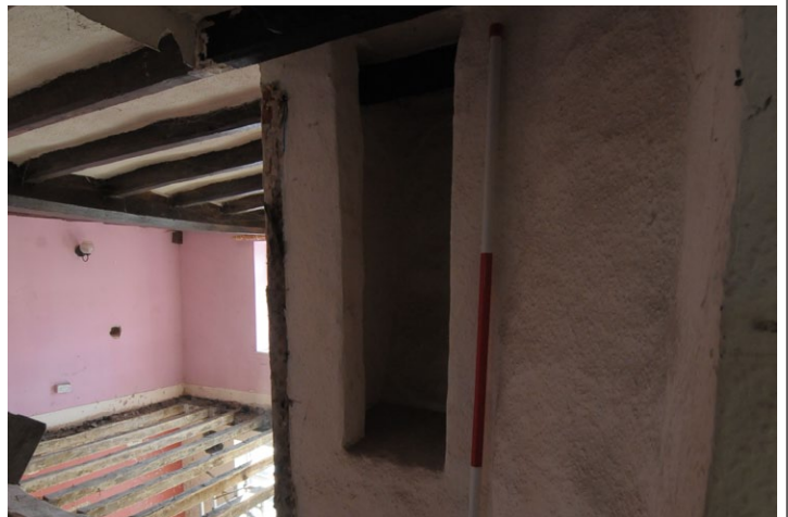
Fig. 22 - Recess in chimney stack, 1st floor, Unit 1, looking south-east
