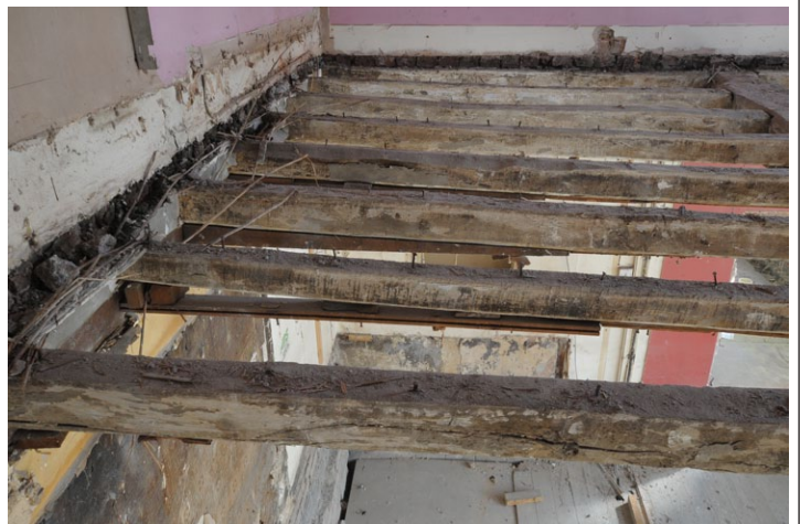
Fig. 24 - Squared floorboard nails in joists, east room, 1st floor, Unit 1, looking east
