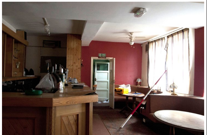
Fig. 12 - Photo of east end of ground floor, Unit 1, looking east
