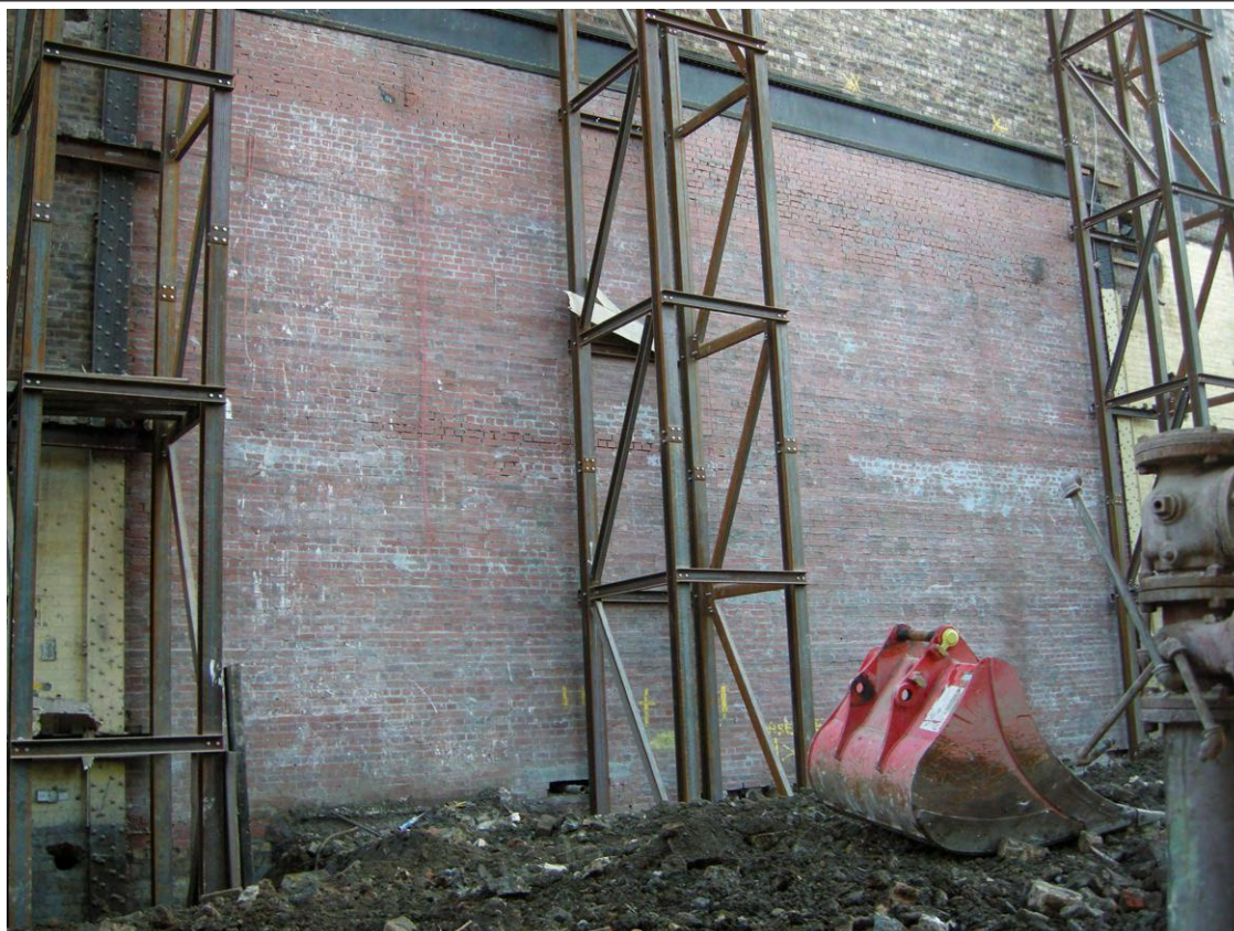
Plate 1 - Exposed wall of the Odeon Cinema with modern infilling between the 1930 rivetted steel frame
