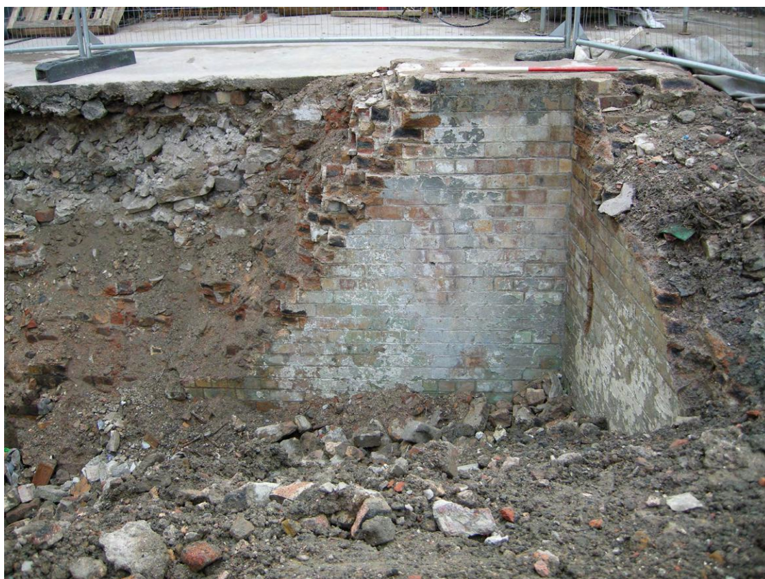
Plate 4 - Area 3 showing the depth of the fly tower basement walls and made ground behind
