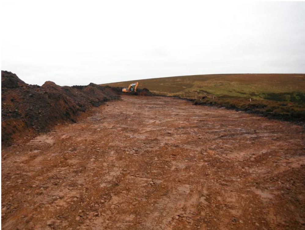
Fig. 5 Final topsoil stripping at Borrow Pit C.
