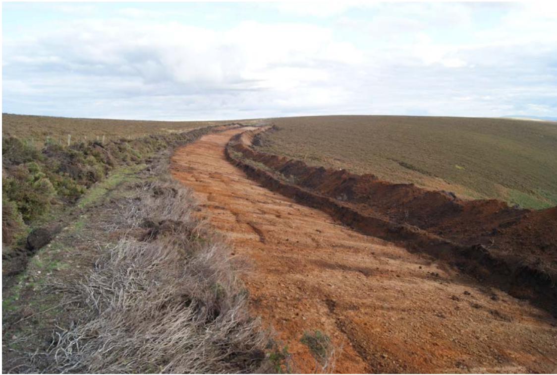
Fig. 4 Access track between Turbines 10, 14 and 16 stripped
