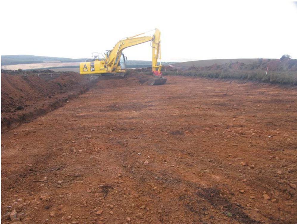
Fig. 6 Final topsoil and subsoil stripping at Turbine10
