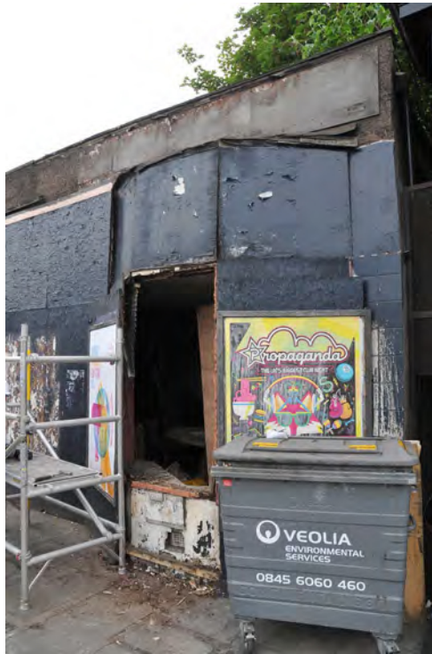
Plate 3: Oblique view of bay window, No.15 Dalry Rd
