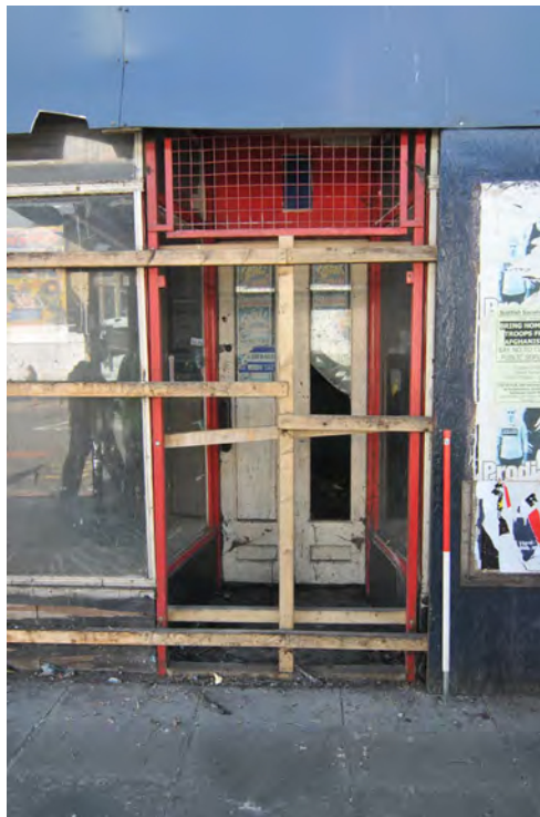
Plate 6: Detail of recessed entrance of No.11 Dalry Rd
