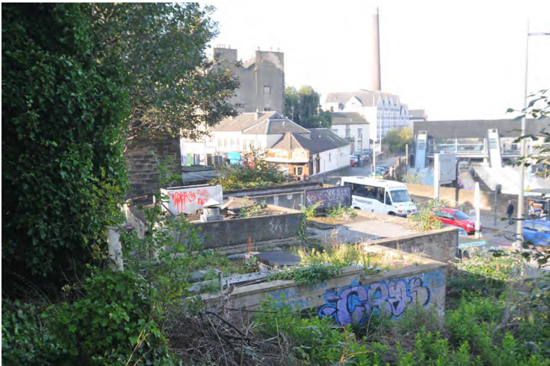
Plate 8: View of roof in setting from the north-east
