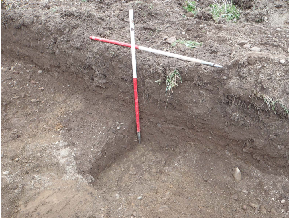
Fig. 8 - Feature 004 in Tr. 4 from the south west
