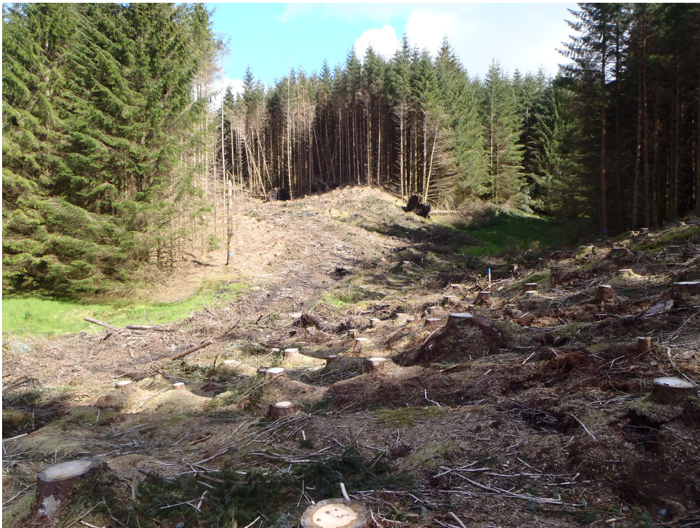
Fig. 5 - Western part of section 1 link road, from west
