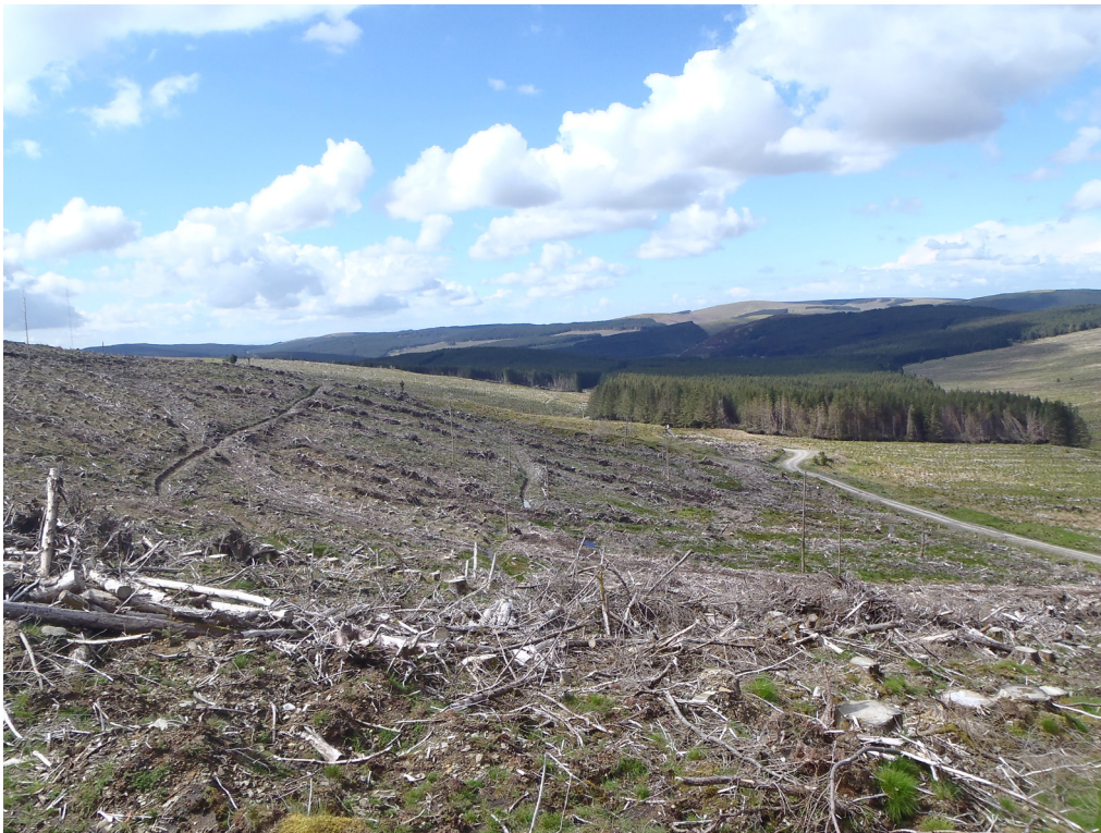
Fig. 3 - Borrow pit H area, from SE
