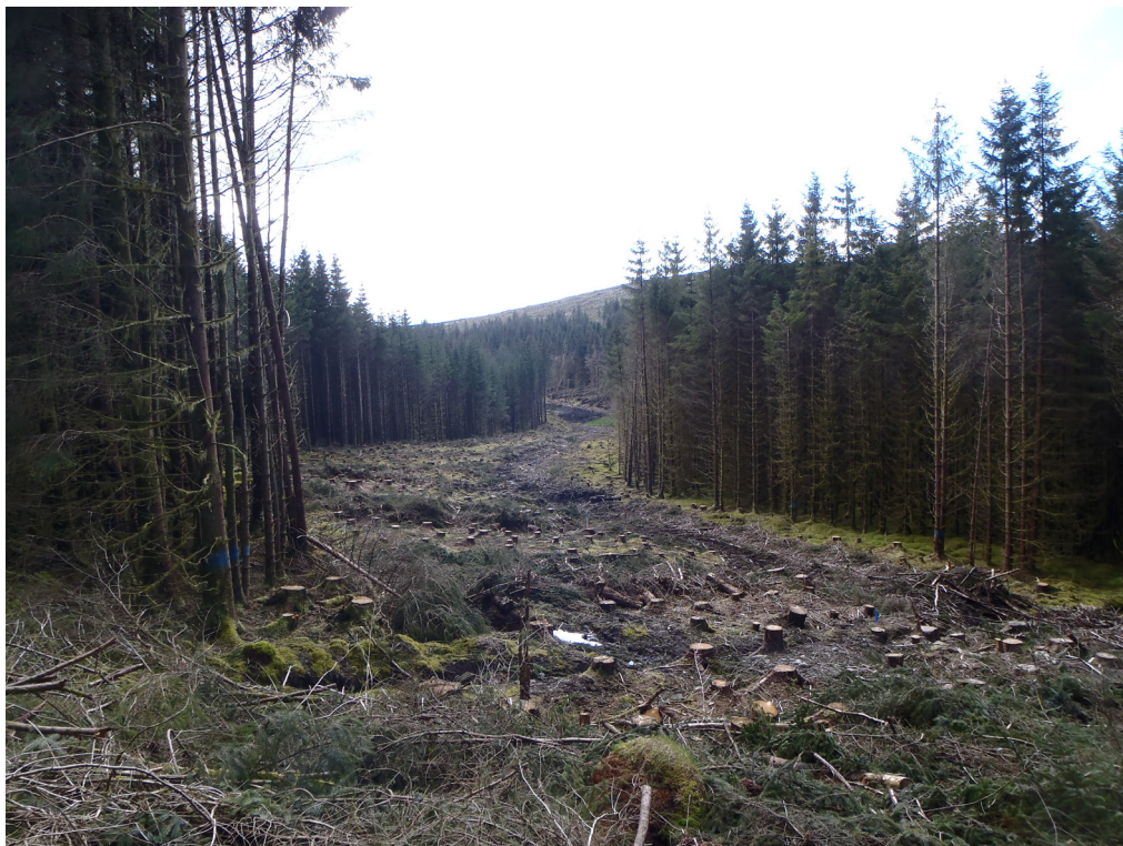
Fig. 6 - Northern part of Section 2 link road, from NE
