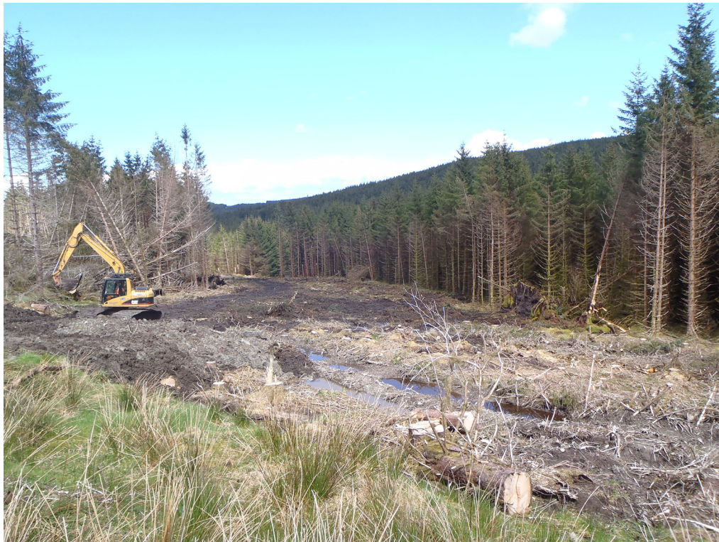
Fig. 7 - Southern part of section 2 link road, from SSW
