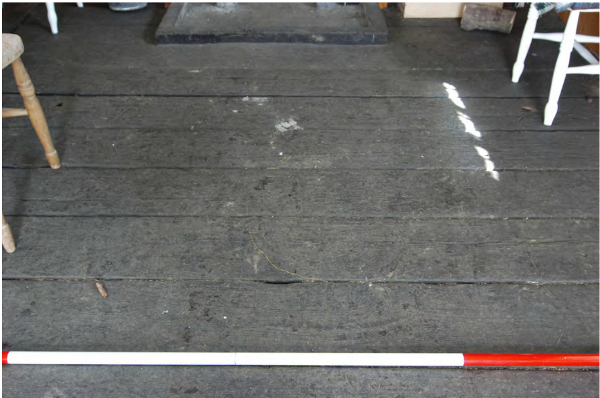
Fig. 10 Floor detail (reused railway sleepers)
