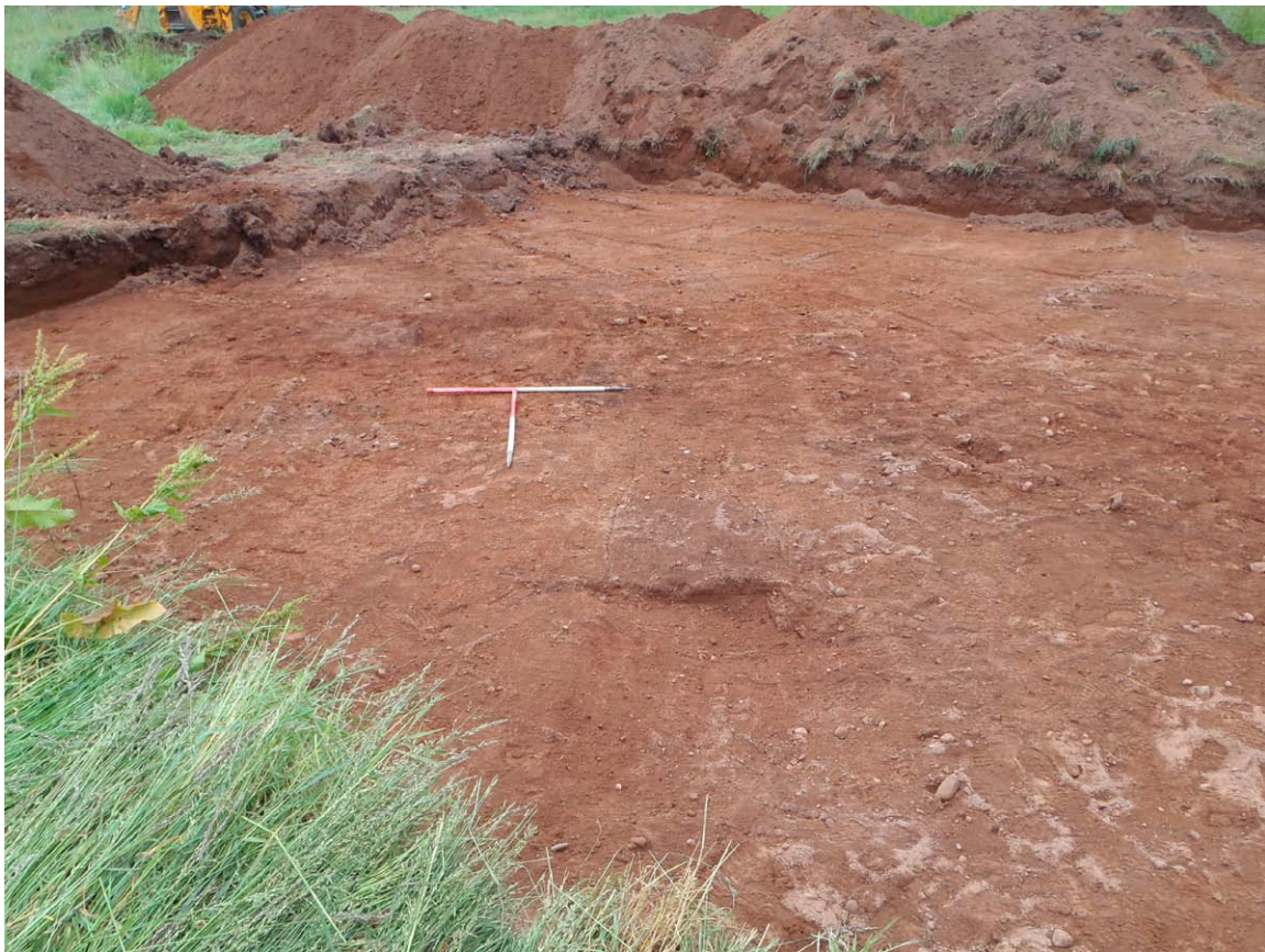
Fig. 6 - Trench 4 showing feature 405, looking South-East
